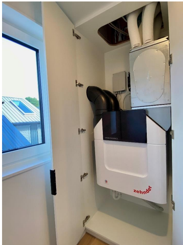
Photo: Ventilation unit within laundry cupboard
