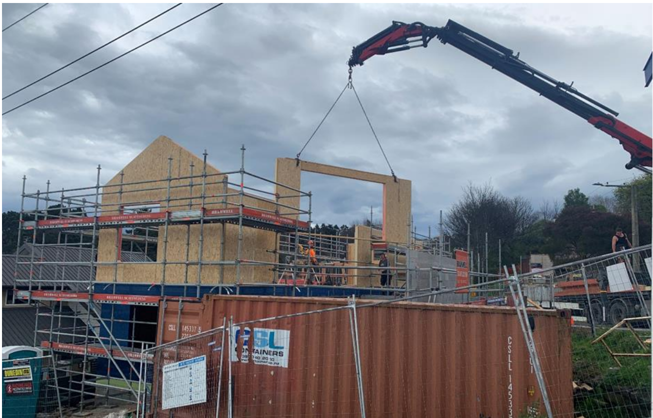
Photo: SIP panel installation
