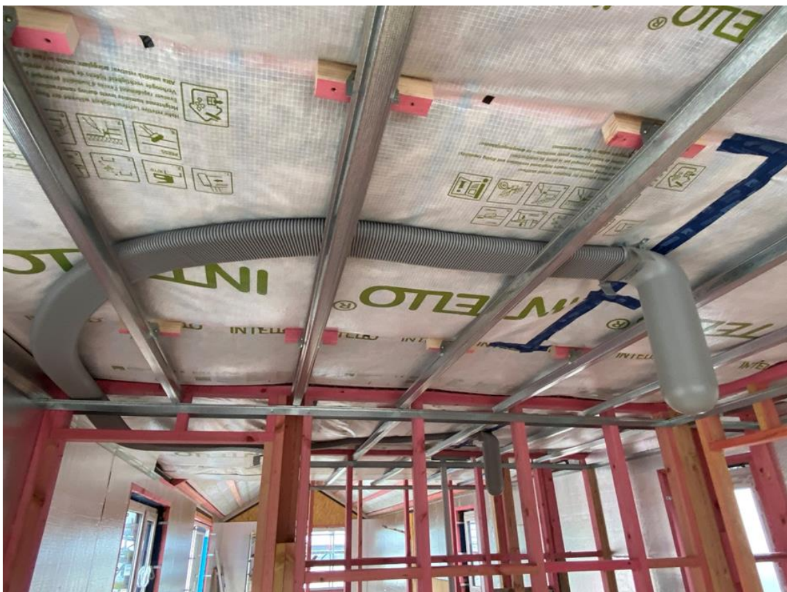
Photo: Ventilation ducting installation
