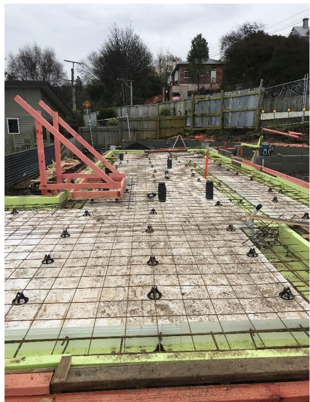
Photo : Concrete Slab Insulation
