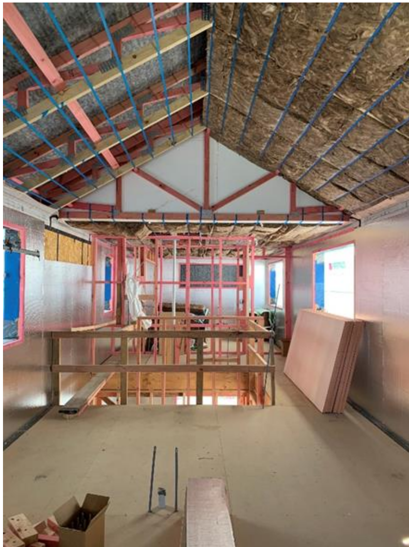
Photo: Roof insulation being installed
