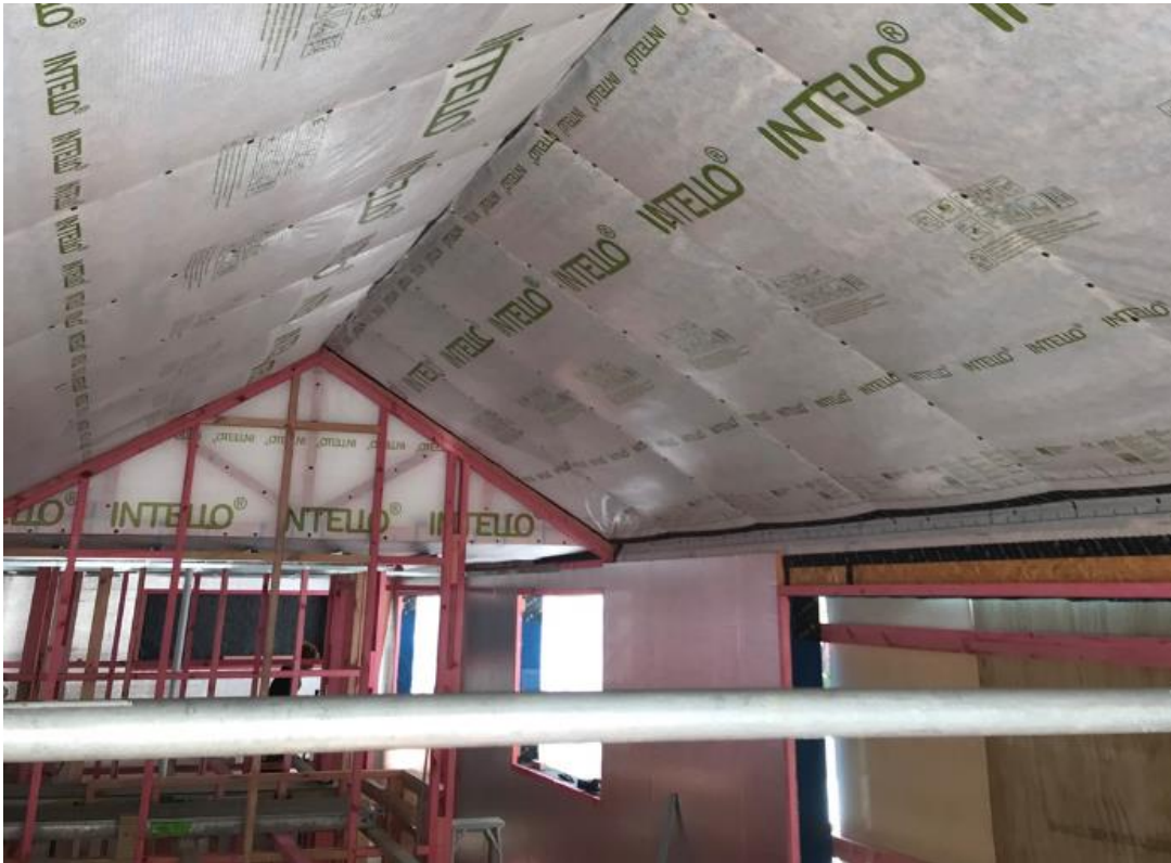
Photo: Airtightness control layer
