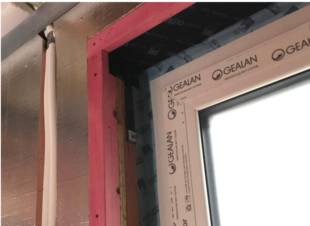
Photo: Air tightness tape to windows
