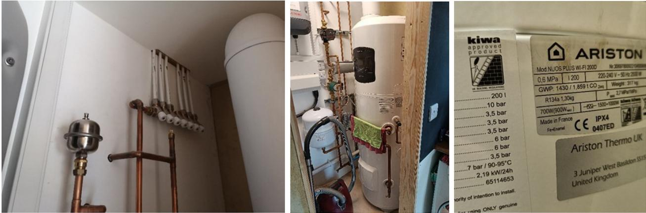
Heat supply is via an Ariston Nuos Plus Air Source Heat Pump with integral hot water cylinder (200l). This is mainly used for domestic hot water but also serves two towel radiators located in the bathrooms (one on each floor). The heat pump is located internally within the plant room, adjacent to an external wall for air intake via direct ducting.
