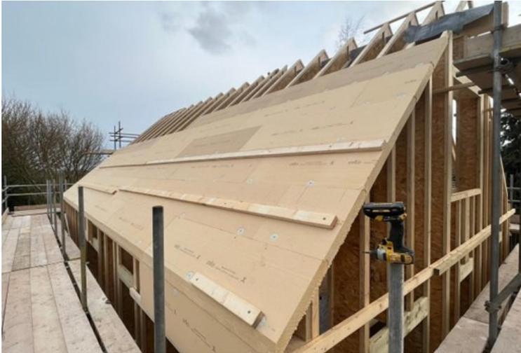
Both the wall and the roof are constructed from 300mm deep timber I-joists filled with Warmcel insulation (blown cellulose) with 80mm wood fibre insulation (Steico Special Dry) and timber cladding on battens applied externally. Internally, 12mm Pro-Passive OSB, with 40mm wood fibre (Steico Internal) with clay plaster. This enables a thermal bridge free junction at the eaves and verge.
