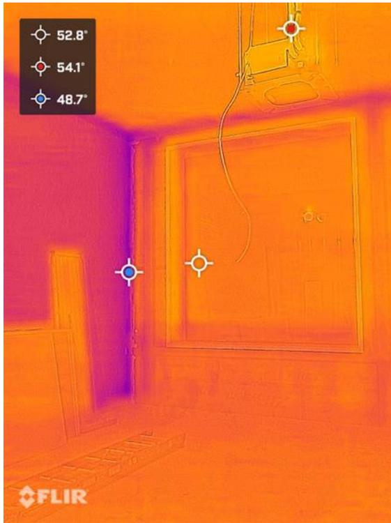
Third floor, NE corner, prior to adding more interior insulation to mitigate thermal bridge at building intersection with neighbor.
