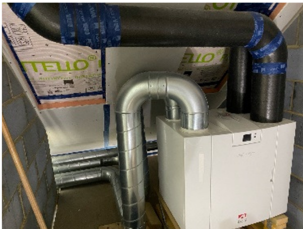
Figure 19. Unit and ducts as installed on site.
