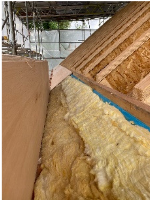
Figure 10. Roof insulation installed on site.
