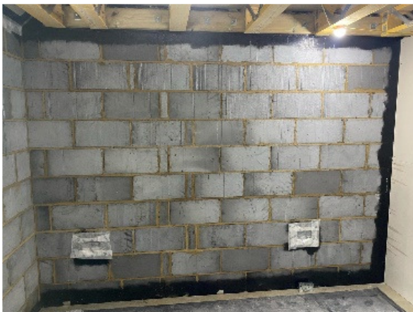
Figure 16. Services airtightness measures.
