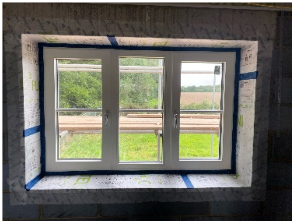
Figure 15. Windows airtightness measures.
