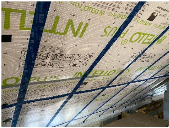
Figure 14. Roof airtightness measures.
