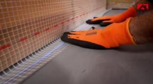
For the connection of the membrane on walls, raise the membrane on 10 cm minimum on the wall and use Colle pare-vapeur Ubbink to make the connection.
