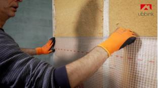
Ensure there is sufficient resistance pressure of the membrane on the frames.
