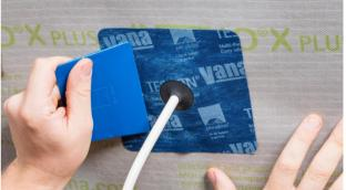
**10a. Joints to cables** Place a KAFLEX cable gasket over the cable and stick to the membrane. The cable gaskets are self-adhesive.
