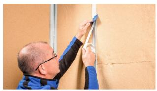
**2. Fasten to stud wall frame members** Fastening of membranes to metal frame members on stud wall and ceiling structures using pro clima DUPLEX.
