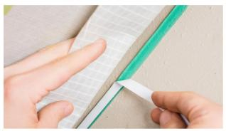
**8a. Alternative: Sealing to mineral subsurfaces** Position ORCON MULTIBOND on the subsurface, roll it out and gradually
