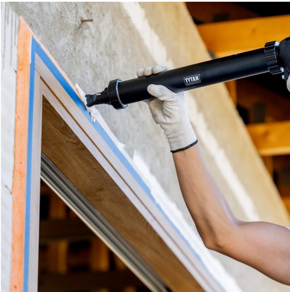
Picture no 15. Application external liquid foils (visible from the outside)
