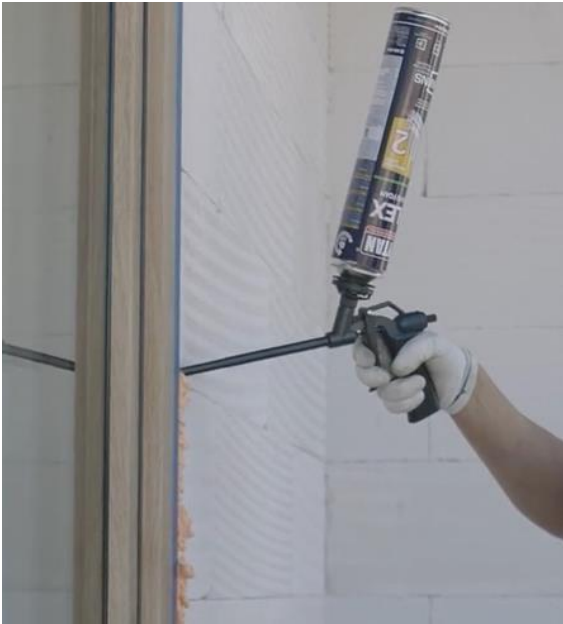
Picture no 7 & 8. Apply the pu foam from bottom to the top from the both sides (visible in the photos from the outside)
