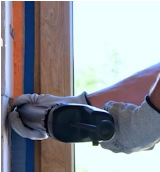
Picture no 17. Application internal liquid foils
