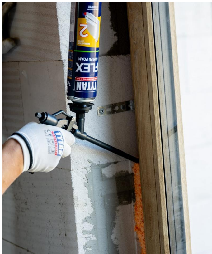
Picture no 6. Apply the pu foam from bottom to the top from the both sides (visible from interior)
