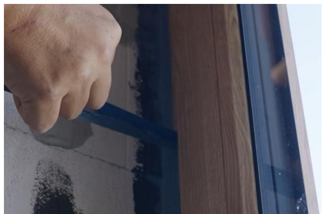
Picture no 18. Removing the masking tape from the inside
