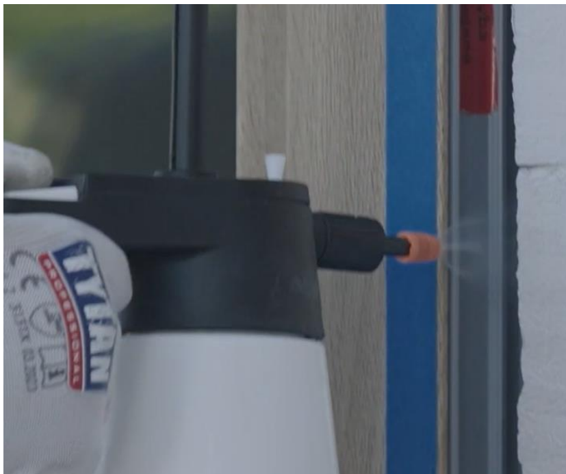
Picture no 4. wet the gap before application by water mist
