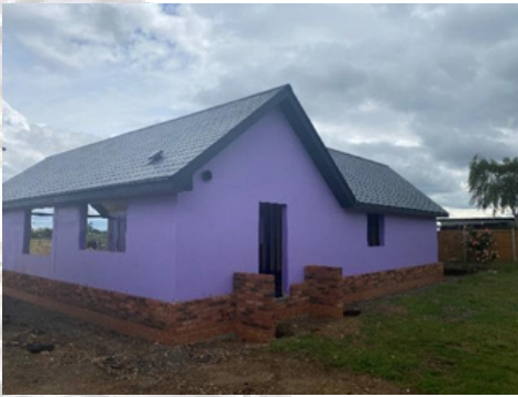
Timber frame install
