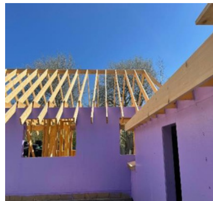
Timber frame install
