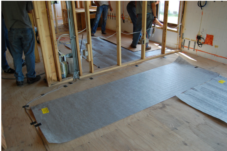
Electric in floor heating mats during installation
