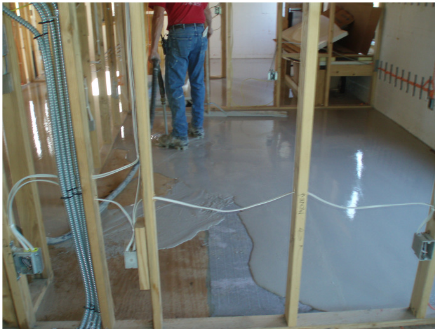
Concrete over-pour on top of electric in floor heating mats
