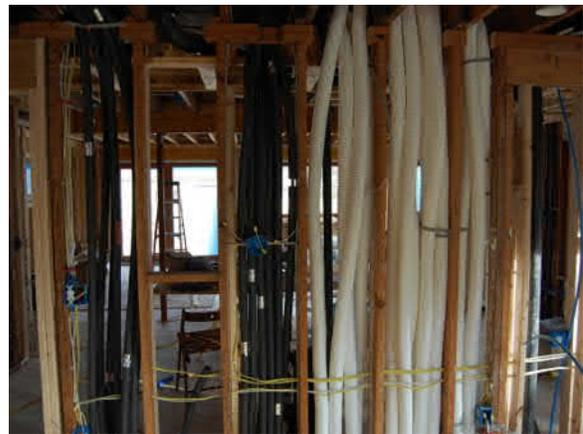
The ventilation system was laid out by TE Studio and commissioned by Zehnder. The ventilation machine offers a summer bypass to maximize passive cooling when available.
