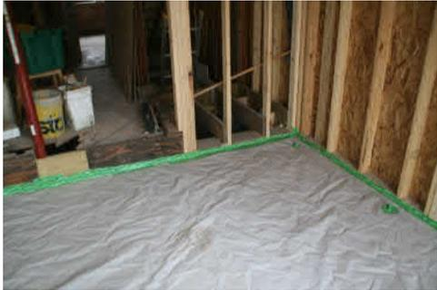
Air sealing at slab
