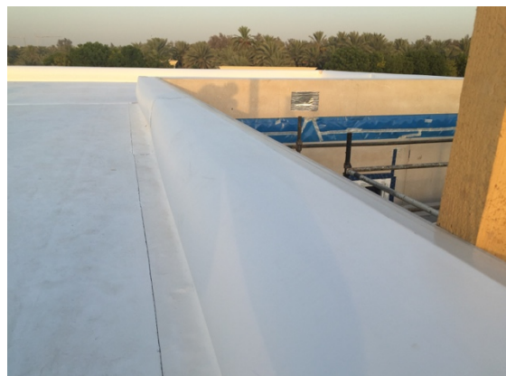
top left and right: XPS over prefab roof bottom left and right: reflective waterproof membrane
