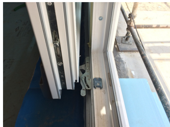
left: pvc frame taped against the vapour barrier before EIFS laying - right: sliding door frames
