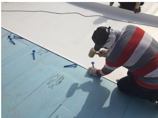
top left and right: XPS over prefab roof bottom left and right: reflective waterproof membrane
