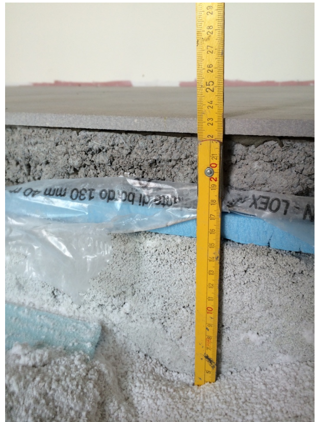
top left: foundations - bottom left: XPS over BV - right: screeds and tiles
