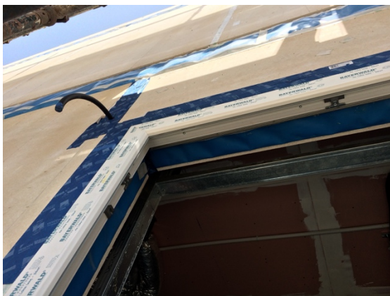
left: pvc frame taped against the vapour barrier before EIFS laying - right: sliding door frames
