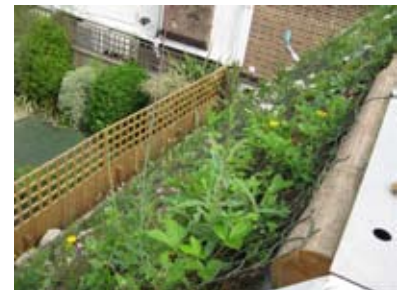
sloping green roof of rear elevation
