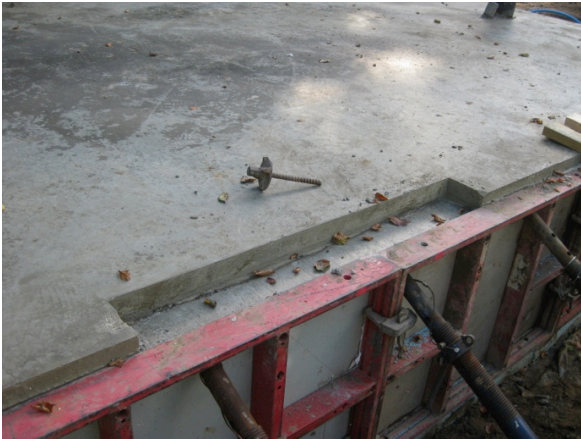
(left) Ground floor door detail, (right) Site photo showing cut in slab for thermal break
