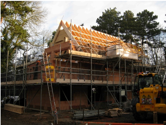
(right) Site photo showing rafters in place
