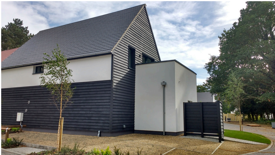
North – limited fenestration, the MVHR outlets and electric meter are visible (Photograph: Sarah Lewis)
