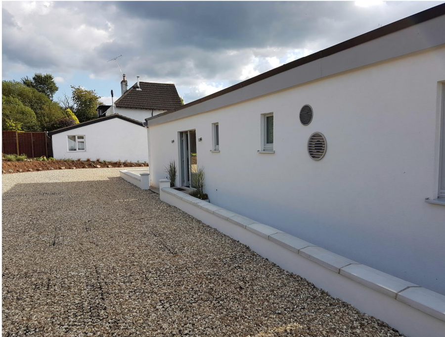
East elevation, the MVHR in- and outlets visible.
