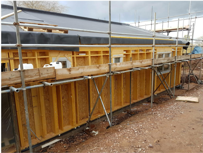
The timber frame before the installation of the insulation.
