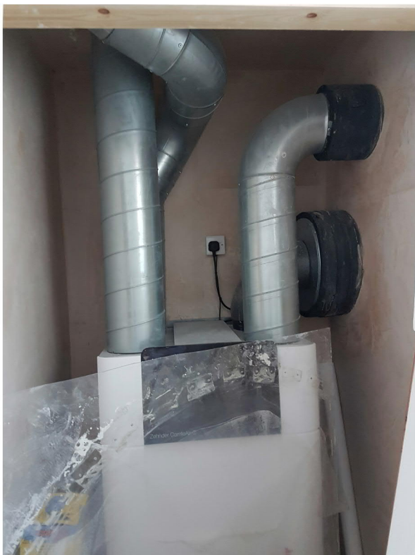
The MVHR and pipework after installation.
