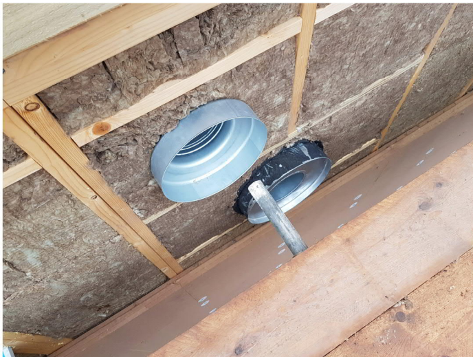
This photo shows the mineral wool fitted between the studs, with the wood-fibre insulation in progress. The pipes are for the MVHR intake and outlet.
