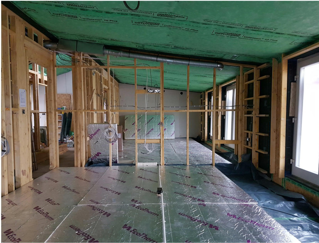
The ceiling with the air-tightness sheeting in place.
