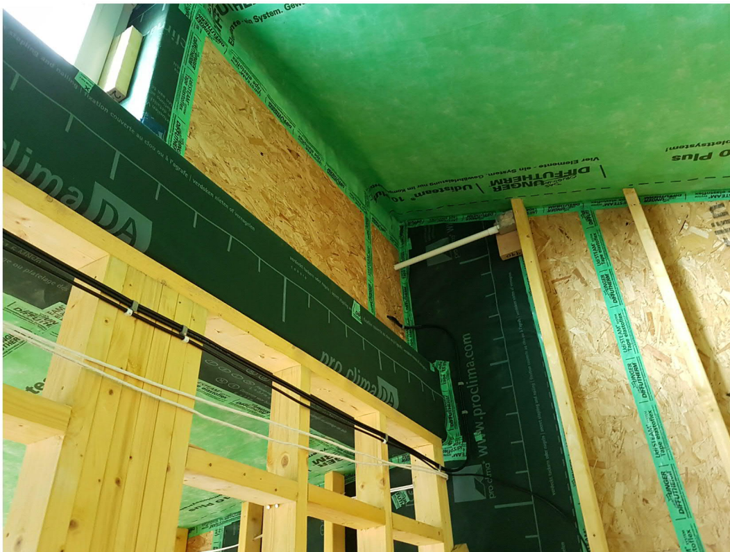
The taping and air-tightness membrane near the clerestorey.
