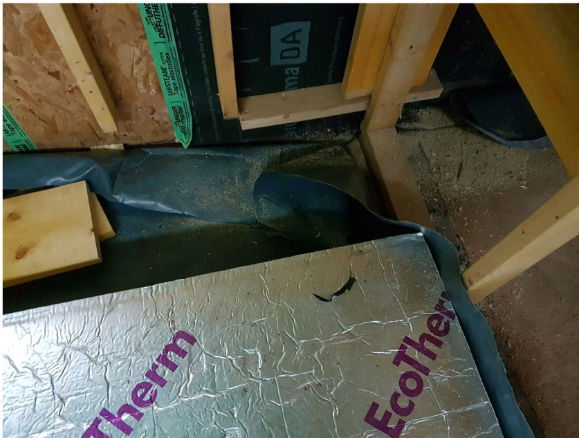
The insulation is being fitted before pouring of the cement screed. The photo shows the junction with internal walls, which were filled with EcoTherm insulation to keep cold-bridging to a minimum.
