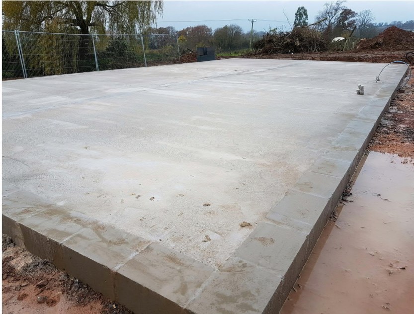
The concrete floor slab the day after it was poured.
