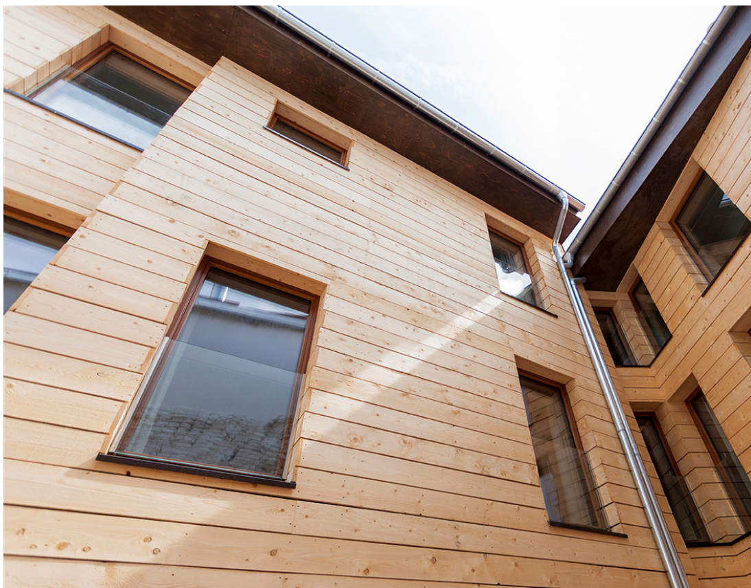
South façade, detail.
