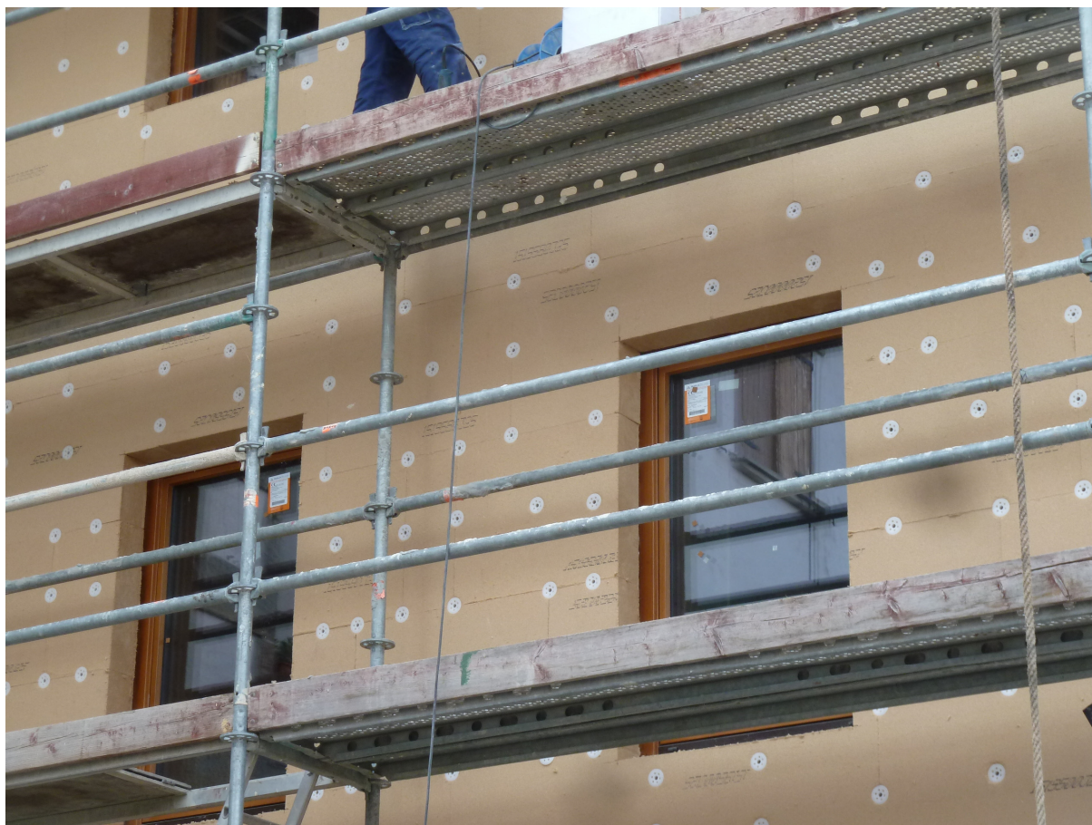
North façade with wood fiber insulation on the brick wall.
