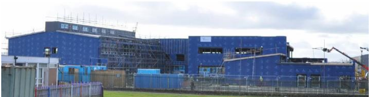
SIPs installation complete and window installation ongoing.
