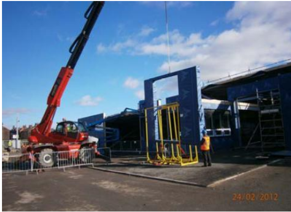
SIPS panel erection February 2012
