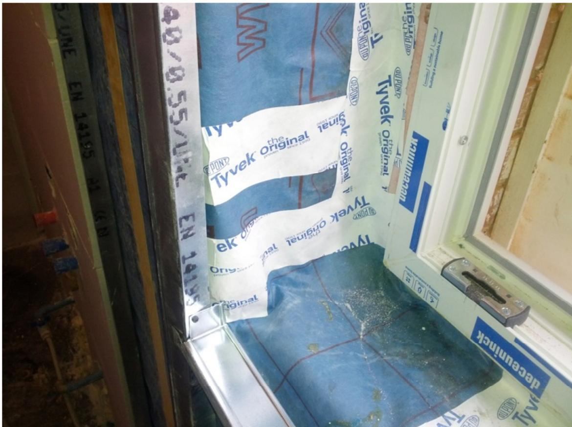
Figure 19: Window-wall airtickness
