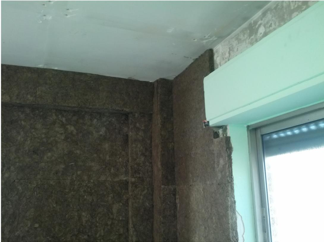
Figure 22: Inner insulation [VAND arquitectura]
