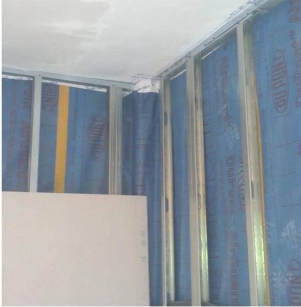
Figure 24: Airtightness layer - PP membrane [VAND arquitectura]
