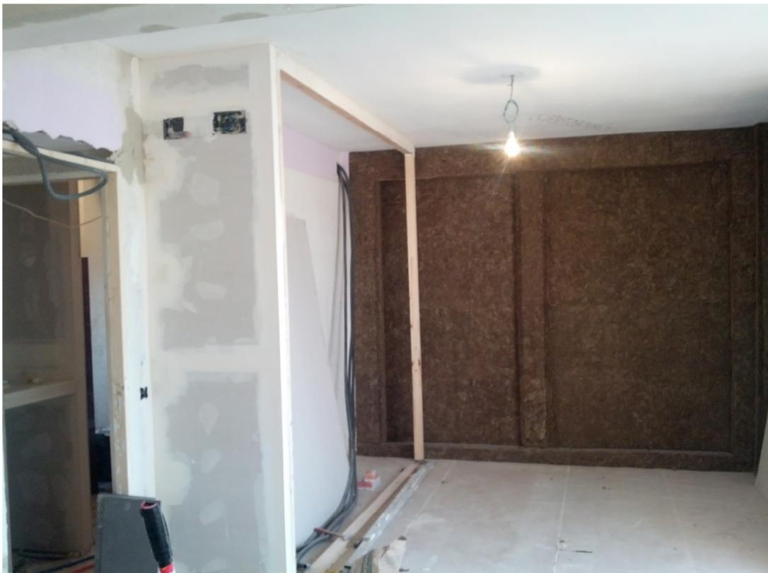
**Figure 21: Inner insulation [VAND architectura]**
