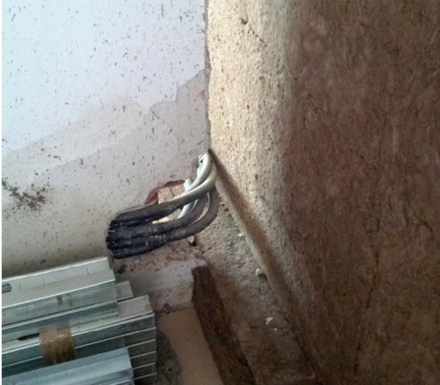
**Figure 20: Continuous inner insulation layer**
