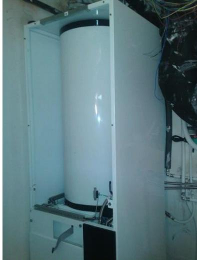
Water-to-Water Heat Pump (Source: DICAM)
