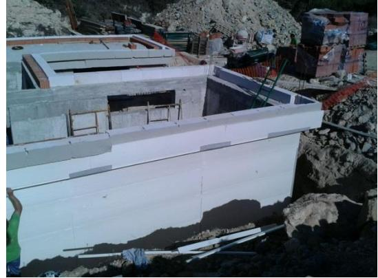
Basement wall insulation (Source: DICAM)
