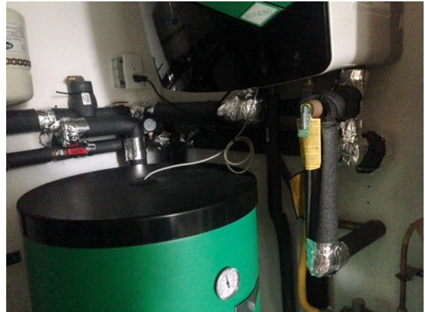
Hot water lines from boiler & storage tank to hydronic coils in HRV
