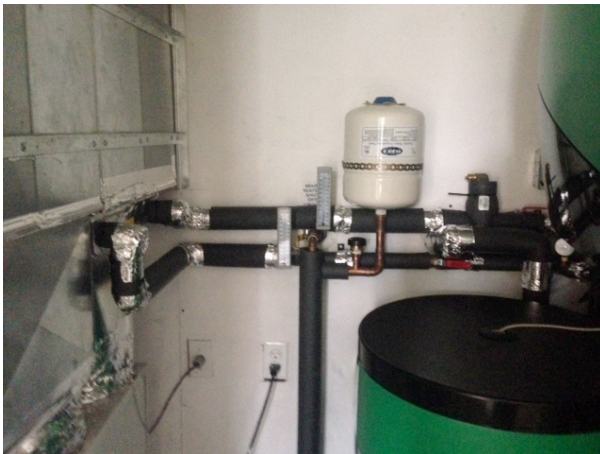
Hot water lines from boiler & storage tank to hydronic coils in HRV
