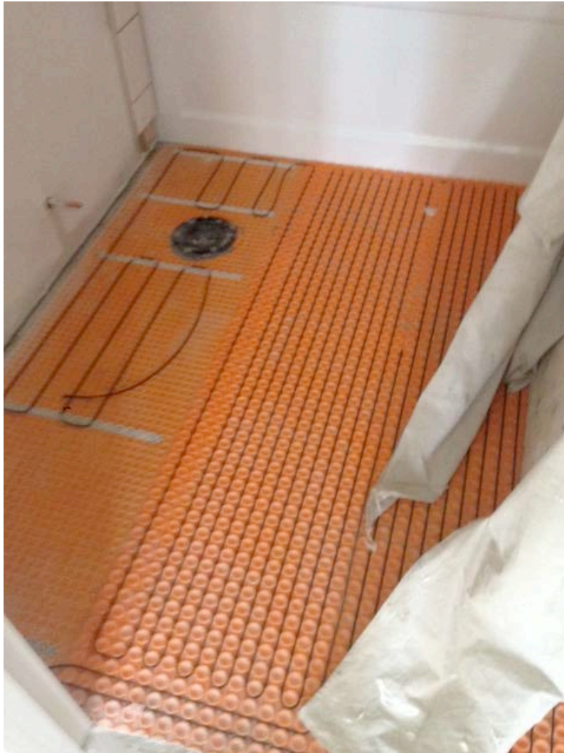
Heat Mat under Bathroom Floor Tile
