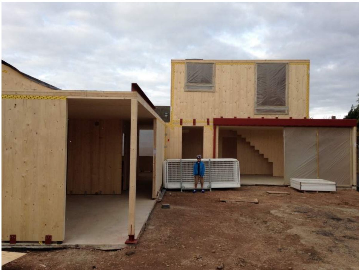
Photo of completed CLT frame
