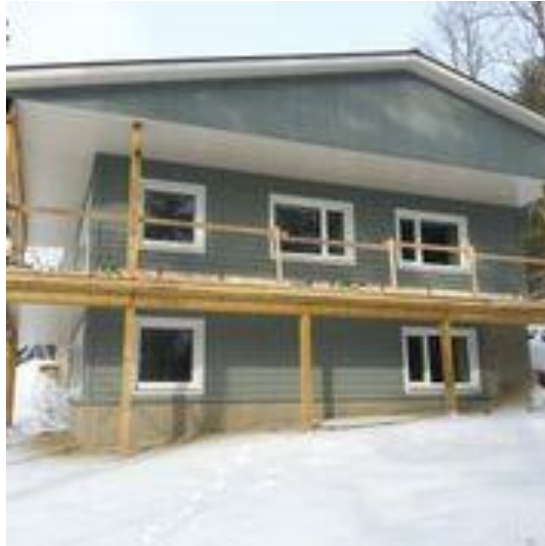
Passive House in Lyndhurst, Ontario, view from the East : showing the deep overhangs and the walk-out basement during construction.
