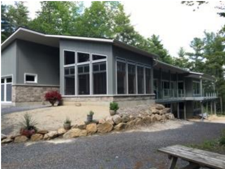
Picture of the Passive House in Lynhurst, Ontario from the Southwest side ; showing the deep overhangs and the walk-out basement.
