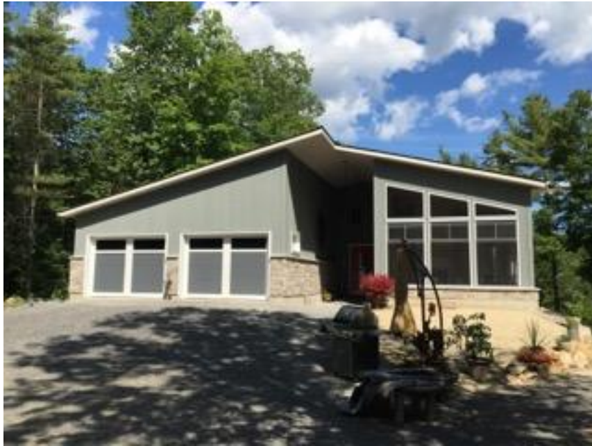
West side of the Passive House in Lynhurst, Ontario with a two-car garage and an enclosed porch that are both exterior of the thermal envelope. (Photograph: Wykes)
