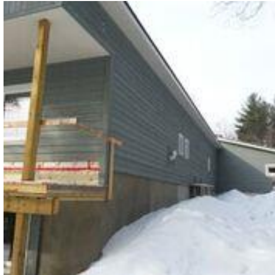
Passive House in Lyndhurst, Ontario, view from the North : showing the depth of grade on this façade, as well as the two condensers for the ductless mini splits during construction.
