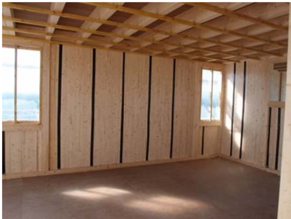
Sealing between panels on the interior with SWS Tape (Soudal)
