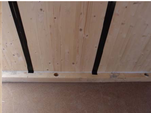
Sealing between panels on the interior with SWS Tape (Soudal)
