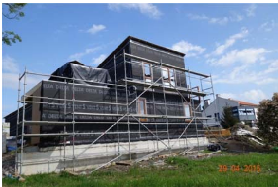
Sealing layer on the exterior of the wooden frame
