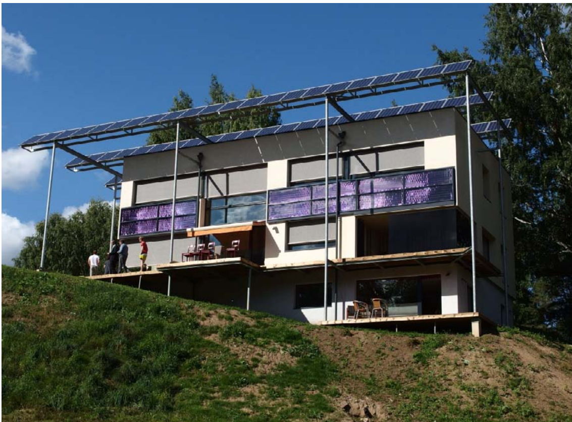
Photo 02.- South and East Facade
