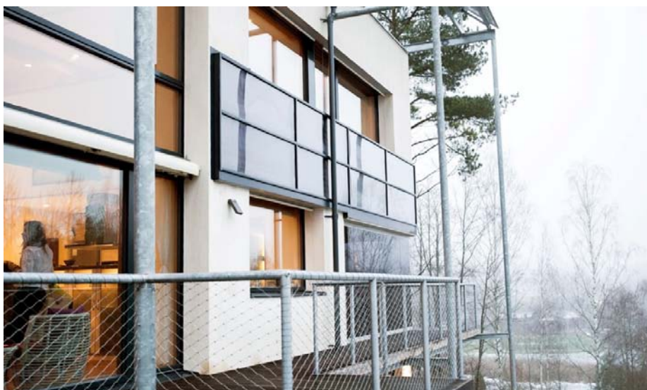
Photo 13.- Hot water collectors, integrated into the facade
