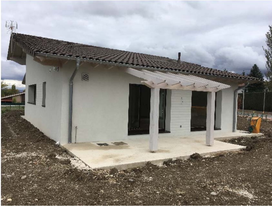
West view, with porch in the foreground
