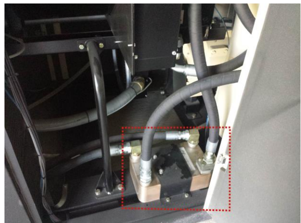
Heat exchanger into compressor's hot air outflow
