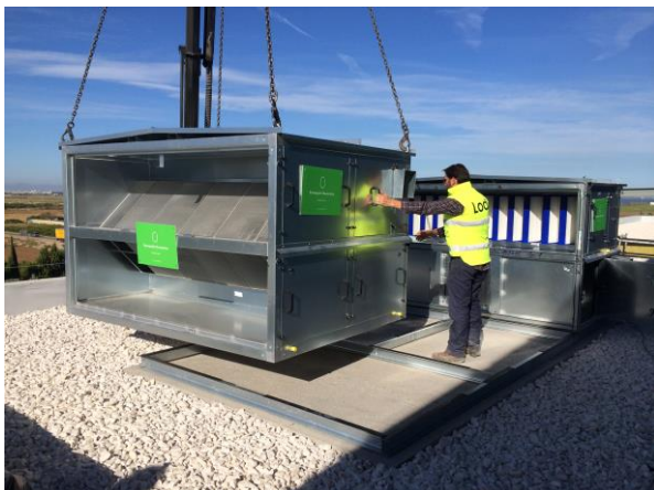
The picture shows the heat recovery and the main ducts on the roof of the building.
