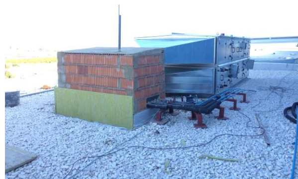
The picture shows the heat recovery and the main ducts on the roof of the building.
