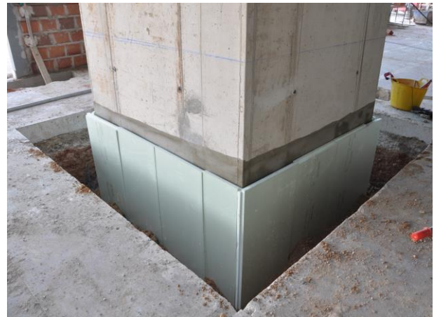
Elevator Core isolation
