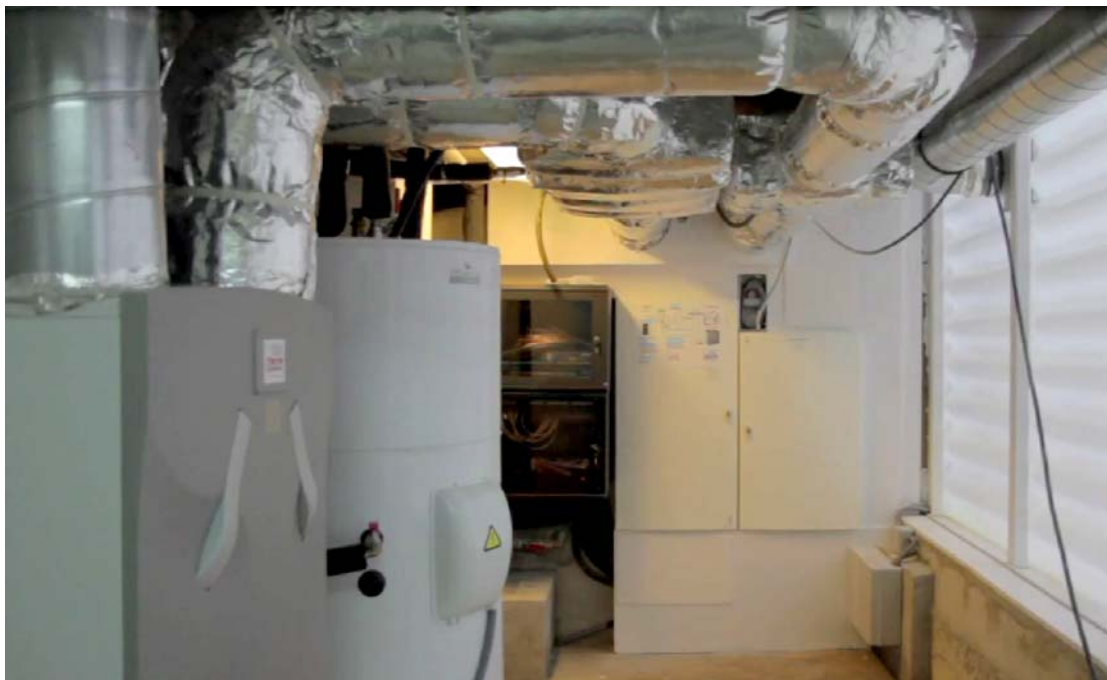
The picture shows the facility room with the heat recovery and the main ducks, and the water tank.
