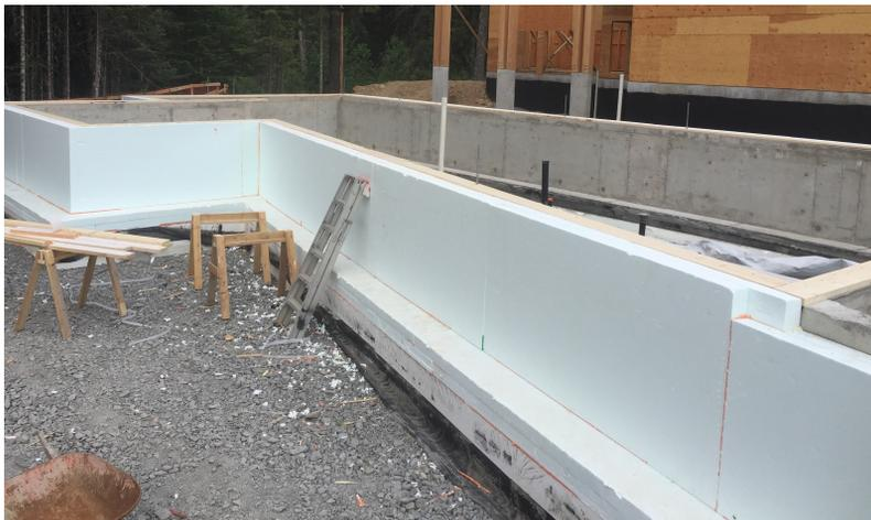
8" (203mm) of EPS wrapped on exterior of footing and foundation wall
