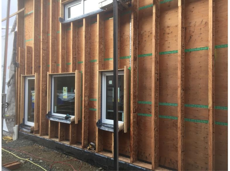
**Interior Airtight Layer (Vapour Control):** foundation concrete, taped plywood (SIGA Rissan), continuous membrane on ceiling (PROCLIMA Intello taped with Tescon Vana)
