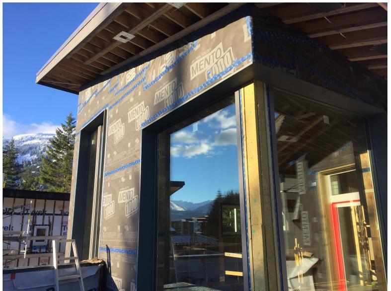
**Exterior Airtight Layer (Water Resistive Barrier):** foundation water proofing (SOPREMA Colphene peel & stick), continuous membrane on walls and sub-roof (PROCLIMA Mento 1000 taped with Tescon Vana), Window sills (GRACE Vicor), Window airtight connection (PROCLIMA Tescon Vana).
