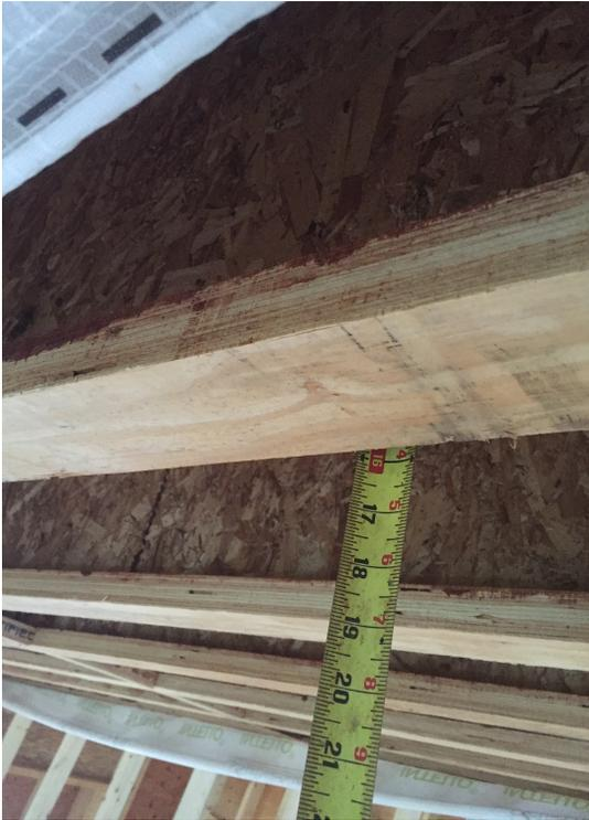
16" (400mm) TJI structure insulated with dense-pack cellulose
