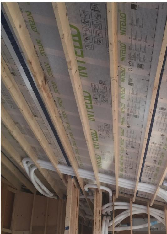
5.5" (140mm) installation cavity insulated with rock-wool
