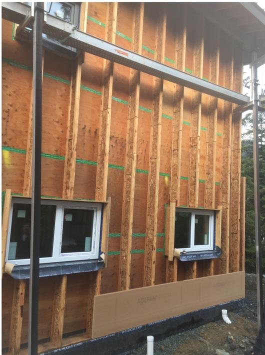
9.5" (240mm) TJI cavity insulated with dense-pack cellulose, 15mm wood-fibre board
