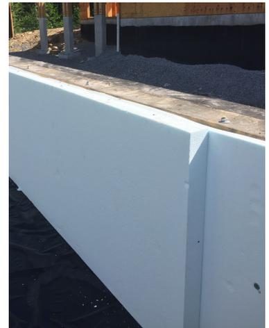
6" (152mm) of EPS on interior of foundation wall
