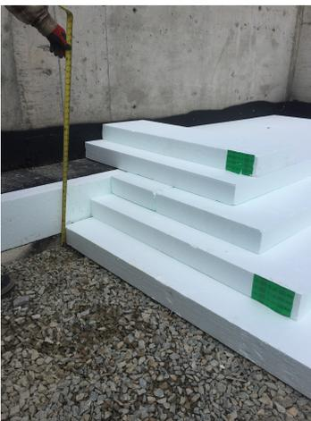
20" (508mm) of EPS under foundation slab
