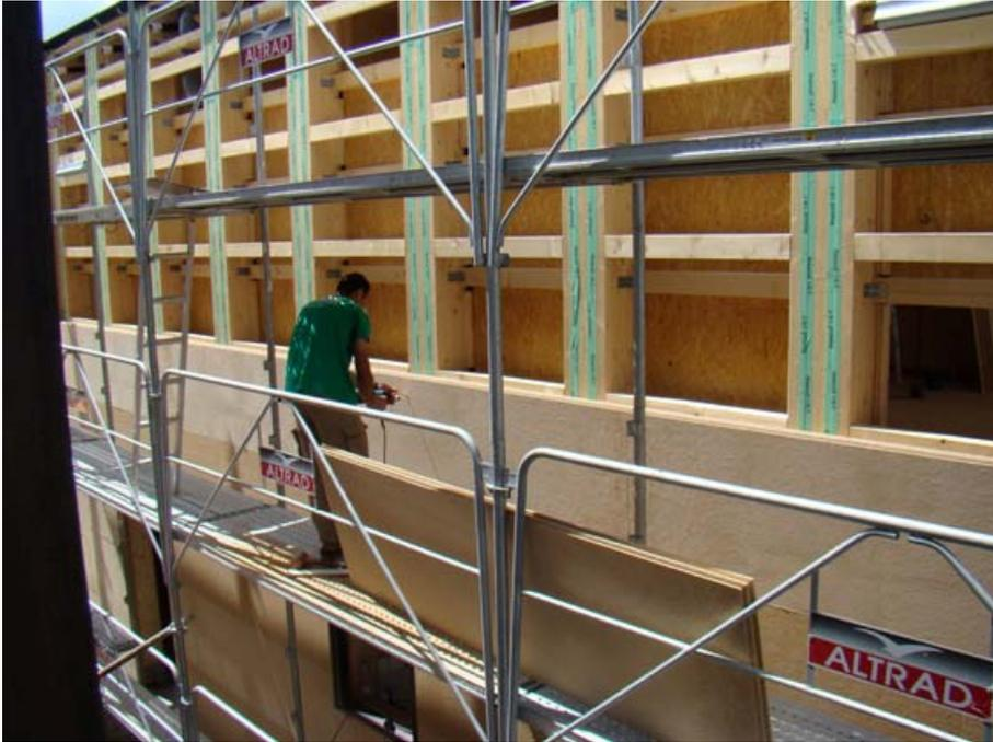
*Installation of the wood-fibre insulation in the outer side of the walls*
