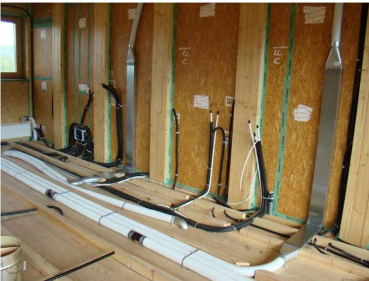
*Ductwork (high density PE) in the floor and in the services cavity (first floor)*
