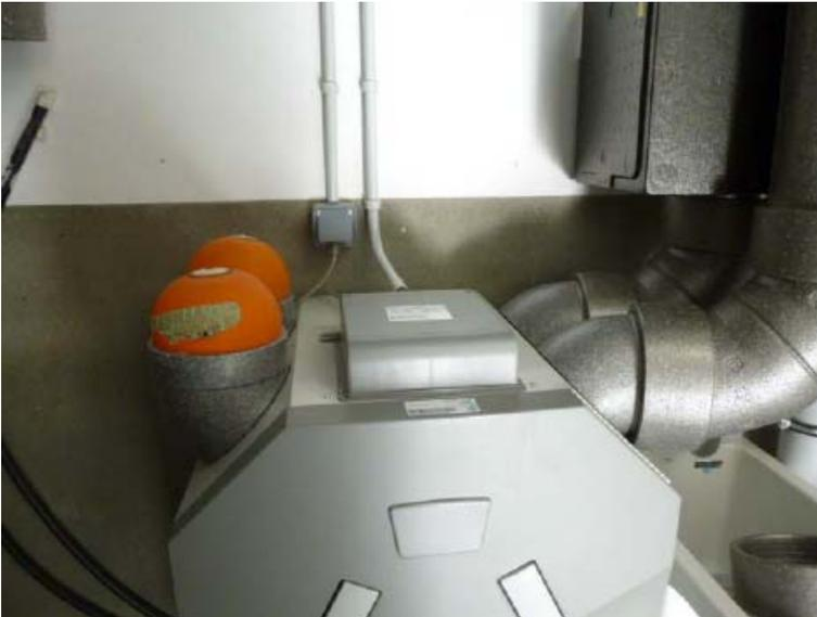
*Provisional sealing of the outside air ducts of the heat recovery unit*
