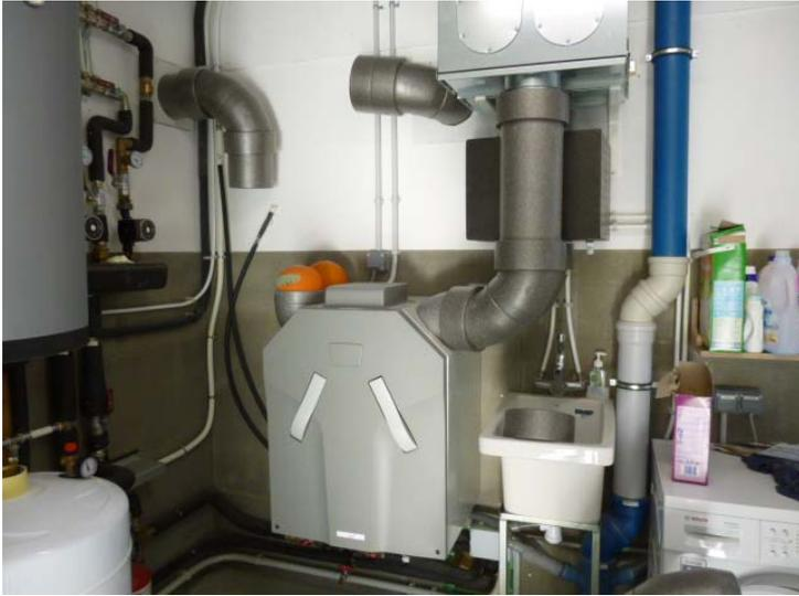
*Heat recovery unit in the garage: photo taken during the Blower Door test: the exhaust and the exterior air ducts are disconnected*
