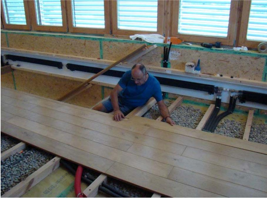
*Floor slab of first floor with gravel to improve summer performance (thermal mass)*
