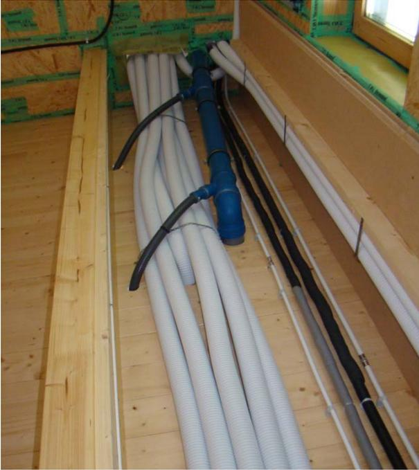
*Flexible duct work (radial system), integrated in the suspended floor section*
