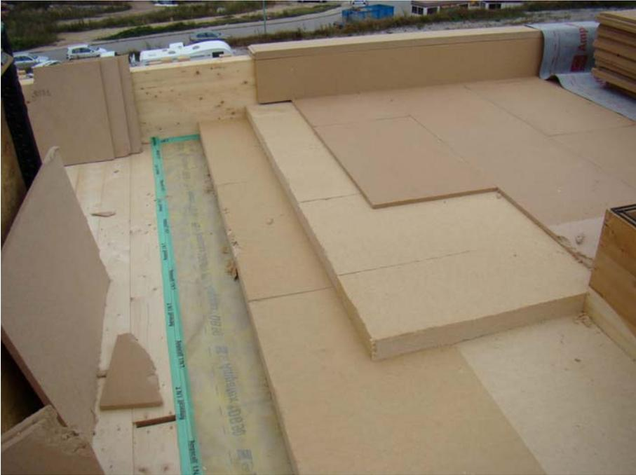
*Installation of the wood-fibre insulation in the roof*
