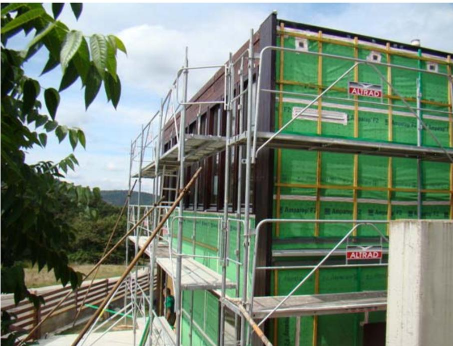
*Installation of the wind barriers for the ventilated facade*
