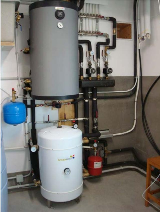
Below: hot water storage tank for heating / Above: storage for DHW
