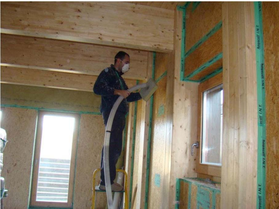
*Blowing in of cellulose insulation*
