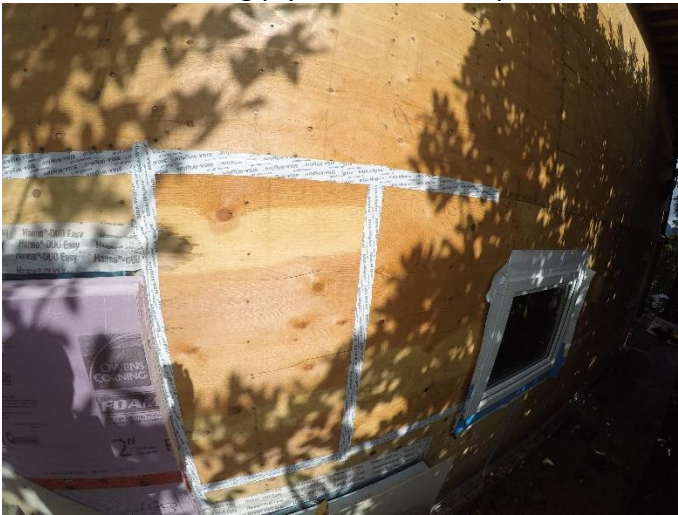
South side showing plywood seams taped
