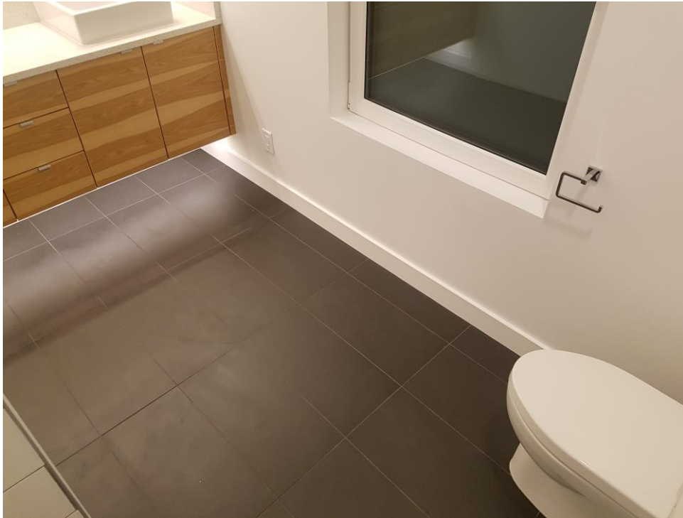
West unit master bathroom tiled floor (heating cables beneath).
