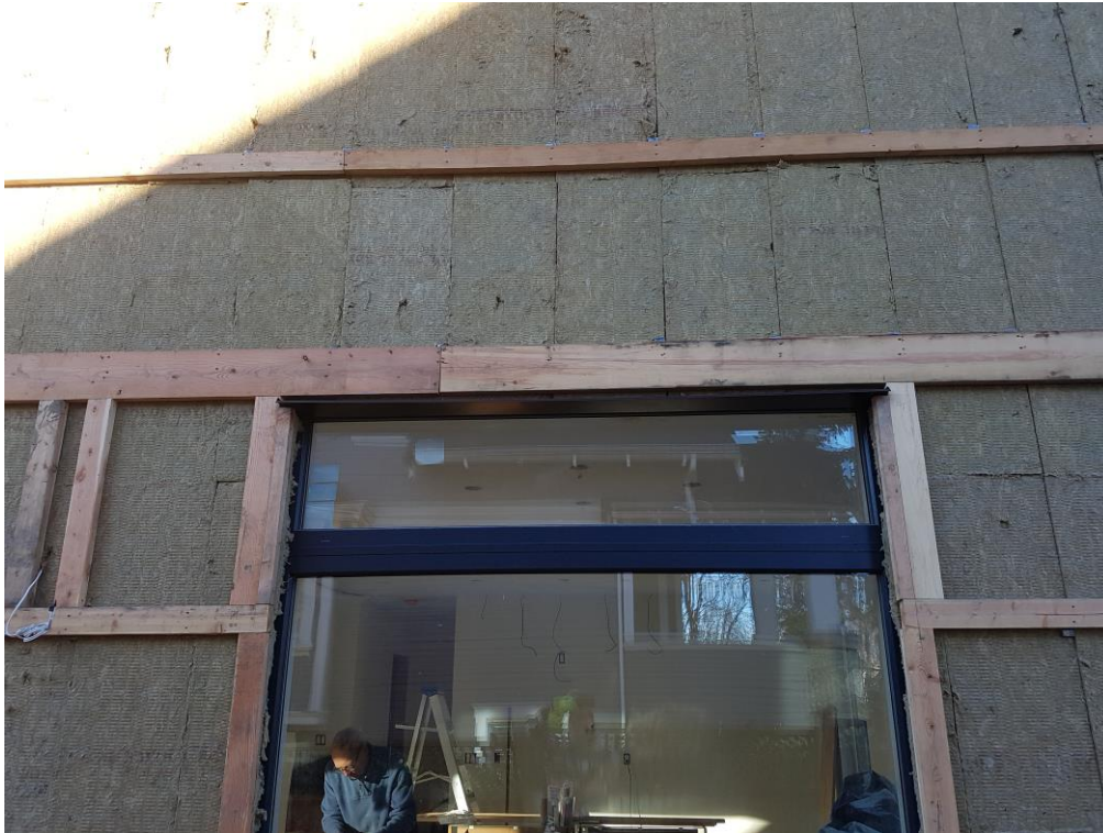
West unit dining room window, pre cladding. Framing around windows protected insulation and provided support from metal window trim.
