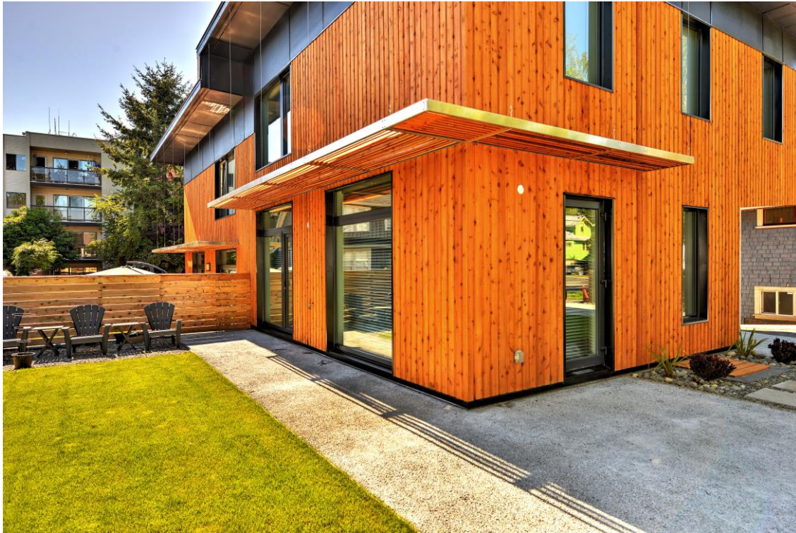
South West; building shading element highlighted. Pervious concrete used for all paved surfaces.
