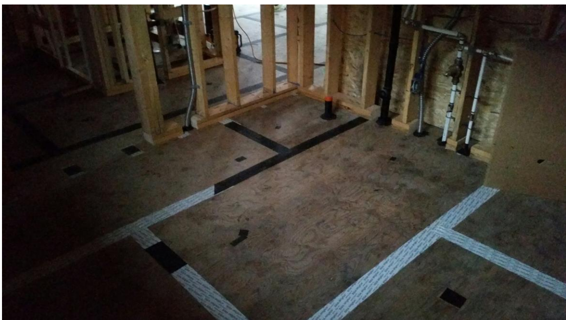
Bathroom floor; penetrations and plywood joints sealed.
