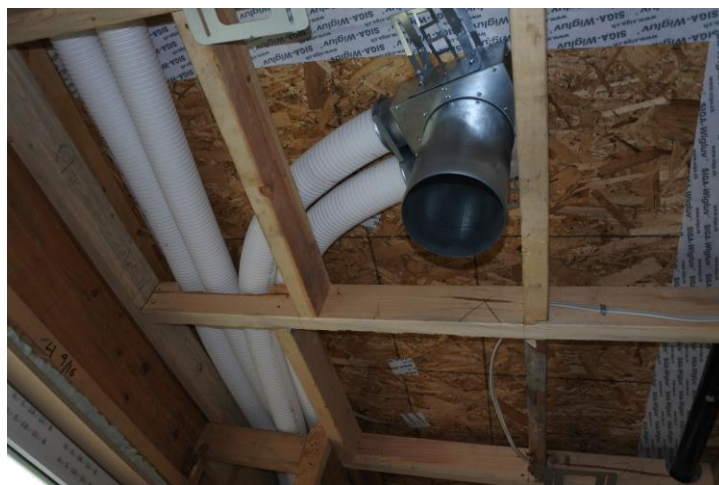
West unit upper bathroom ducting and room connection.
