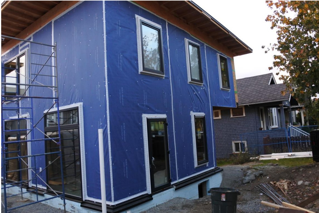
Weather barrier membrane, installed and sealed.
