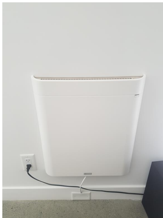
East unit living room wall mounted convection heater.
