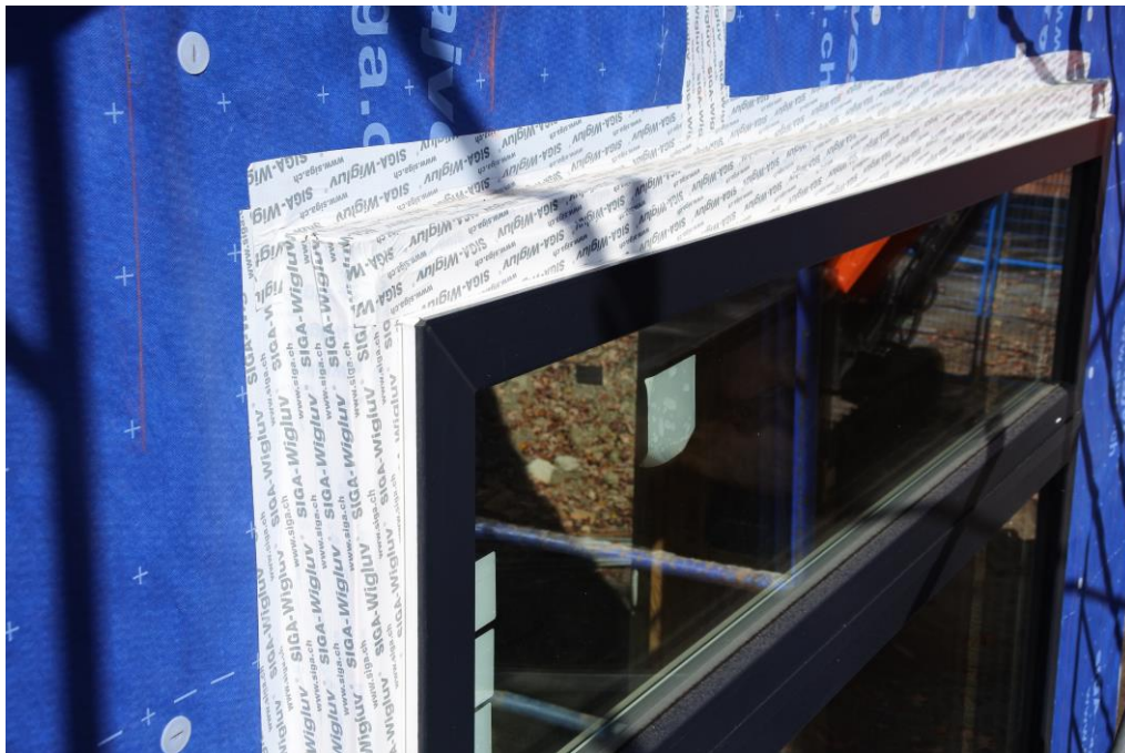
Windows sealed to Siga weather barrier.
