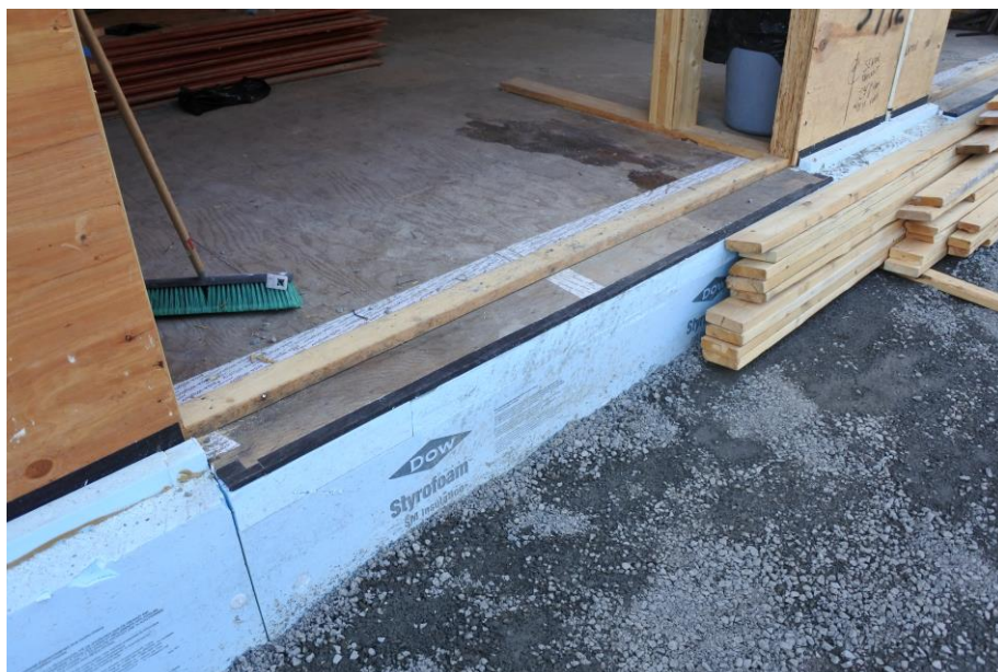
Window sill rough framing at foundation buck assembly.
