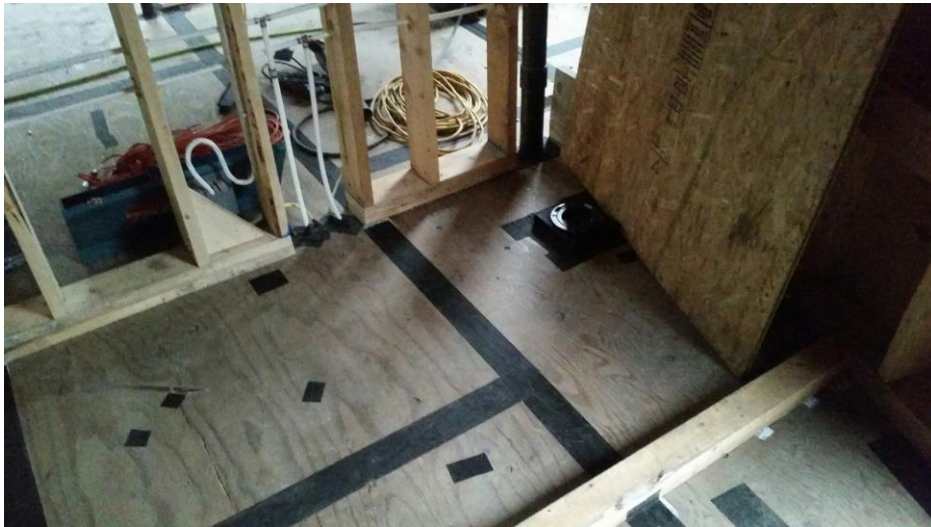
Bathroom floor; penetrations and plywood joints sealed.
