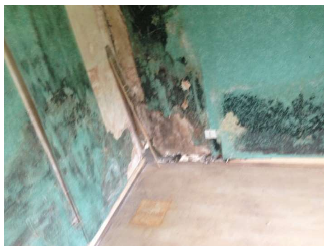
Figure 2 - Moisture between inside insulation and concrete
