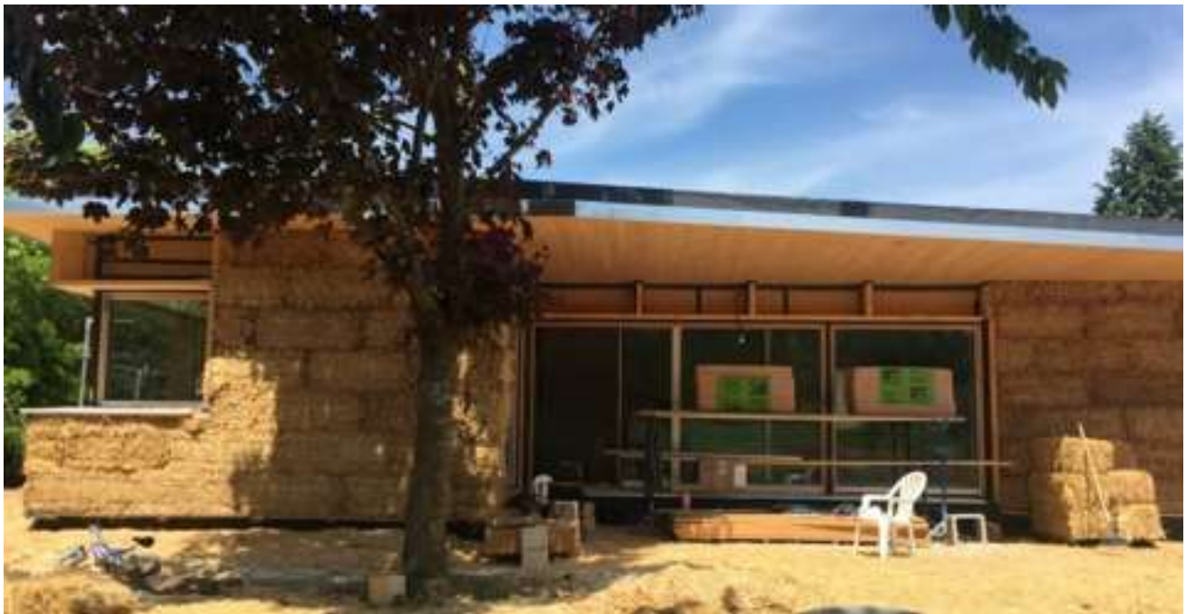
Figure 3 - Straw bale installation
