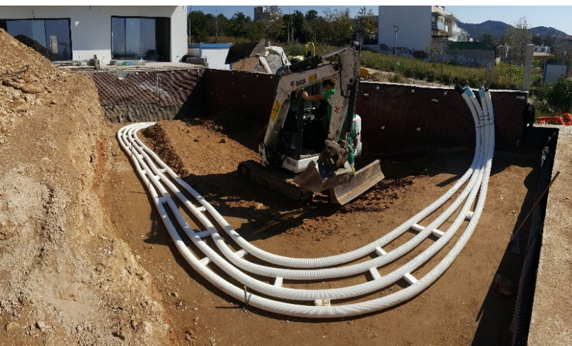
“Pozo canadiense” installation process
