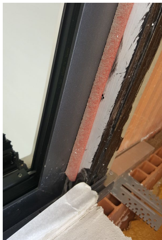
Airtight cover's detail
