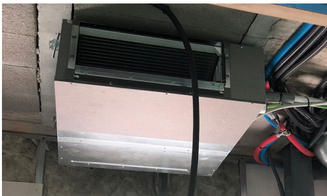
Fancoil for heating and cooling
