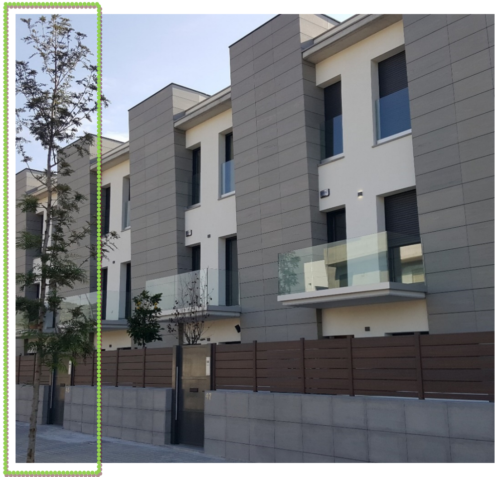
North view of the of the terraced houses, with the certified unity marked in green
