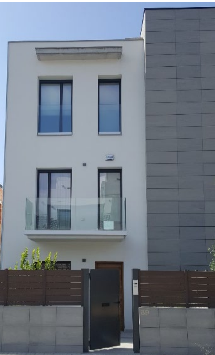
Left: North street façade
