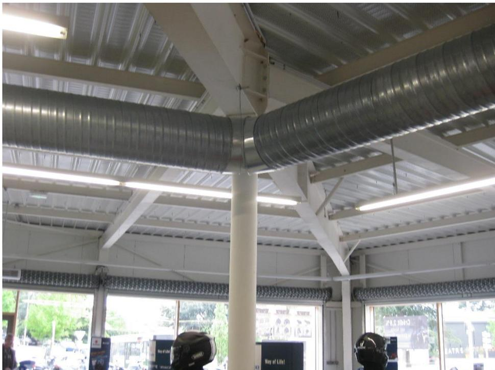
The ceiling includes a white perforated (acoustic), an acoustic vapour barrier, a rock wool and a PVC membrane. It is the best value for money that we have found.
