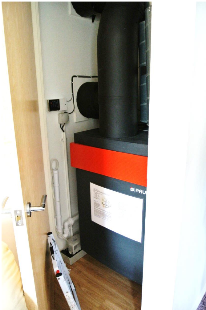
Typical installation of heat recovery ventilation unit.
