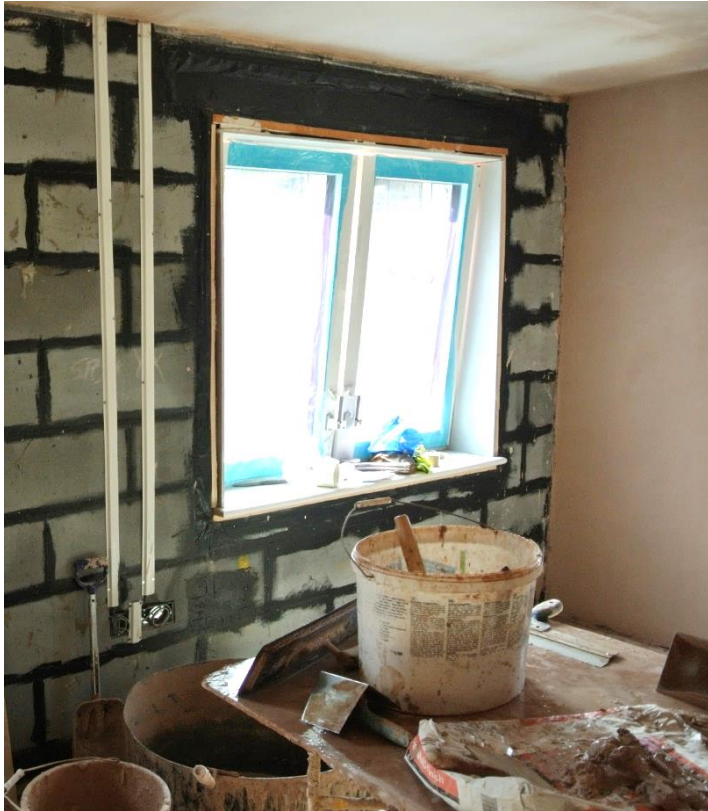
Photo of window installation showing plywood former. Note wet plaster airtightness layer to internal compartment wall between houses and additional Blowerproof airtightness paint applied to blockwork joints and adjacent to the window.
