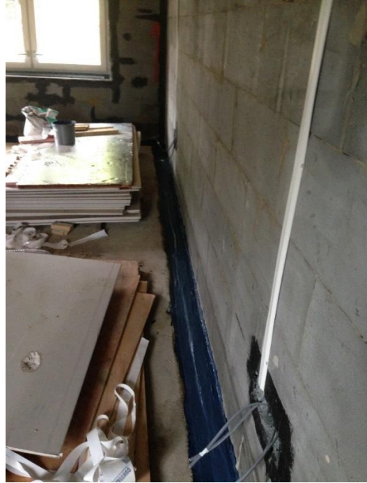
Airtightness – Blowerproof to joints, sockets and windows before plaster applied
