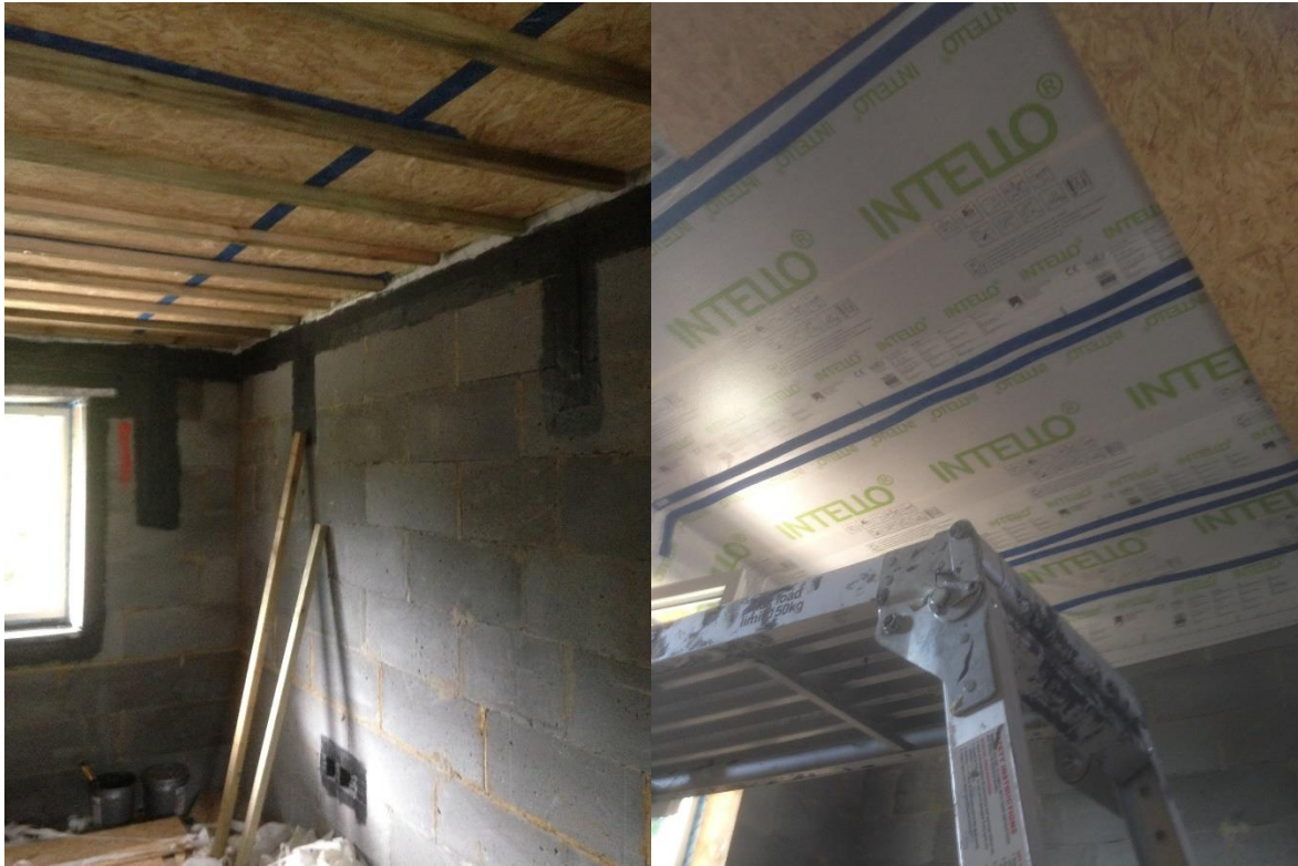
Top floor ceiling installation showing Intello membrane, taped joints, OSB board and taped joints, battens for service void for cables etc.
