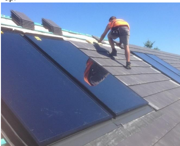
Solar thermal panels during construction – Block 2
