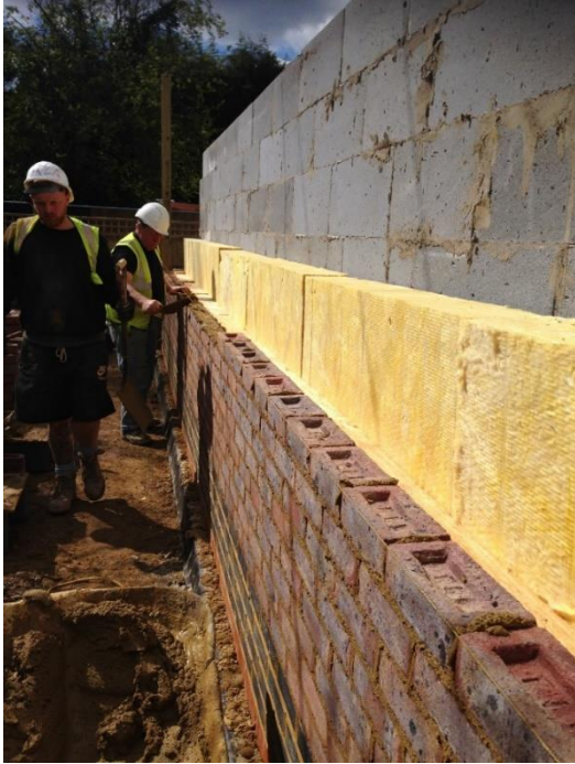
Cavity wall insulation – no gaps
