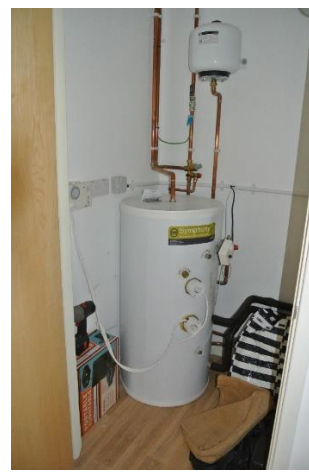
Solar hw cylinder – Block 1 – pipes to be insulated
