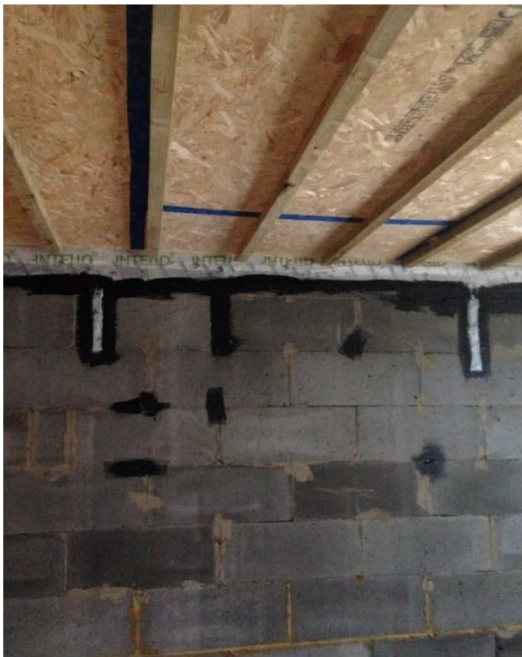
Cavity wall insulation – no gaps
