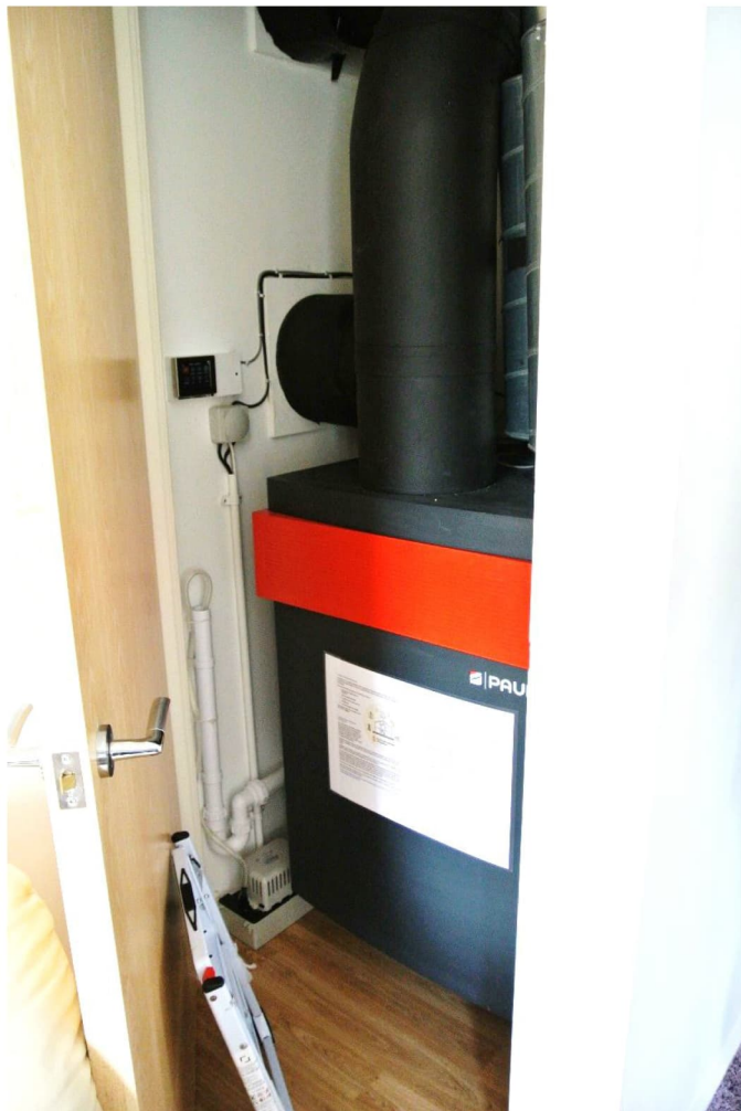
Typical installation of heat recovery ventilation unit.
