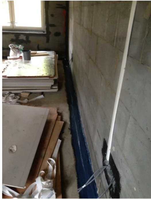
Airtightness – Blowerproof to joints, sockets and windows before plaster applied
