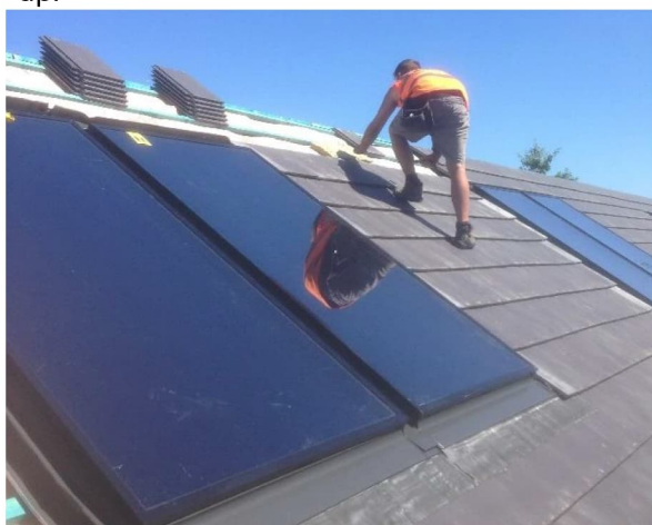
Solar thermal panels during construction – Block 2
