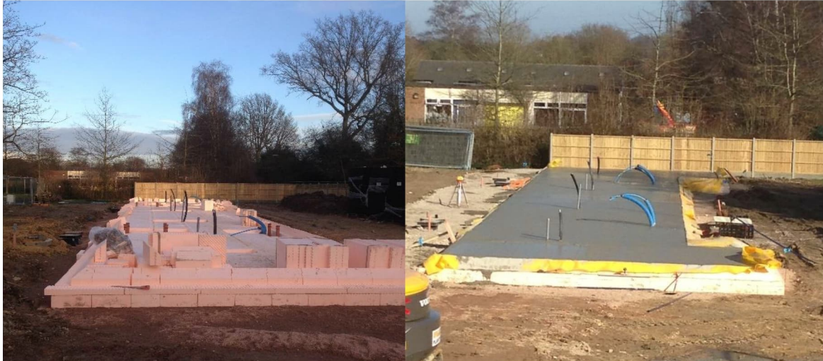
Block 2 insulated raft foundation before and after concrete was poured
