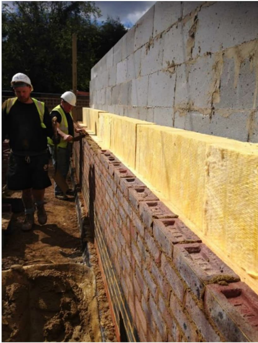
Cavity wall insulation – no gaps
