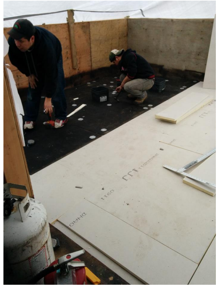
Roof insulation (isoboard)
