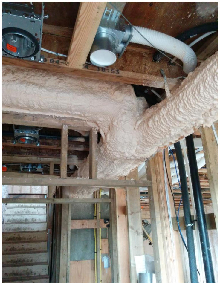
HRV supply and exhaust insulated
