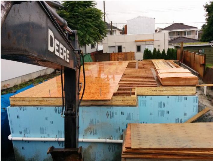
Basement ceiling framing
