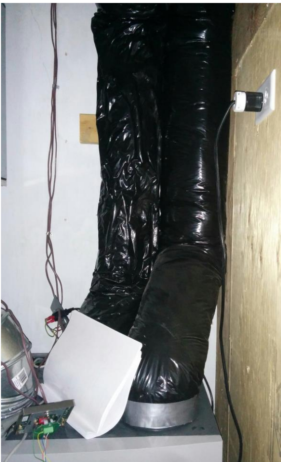
HRV final insulation (only 2m)
