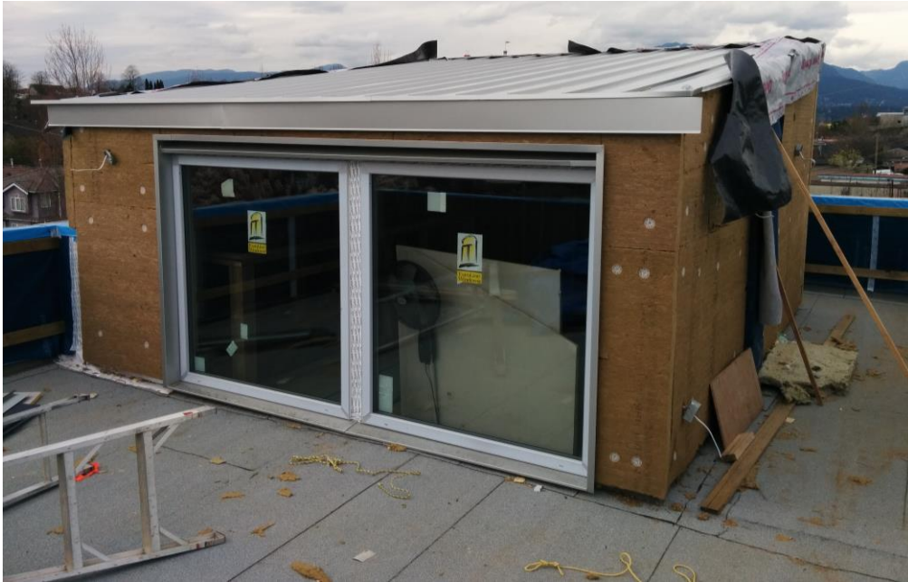
Top roof insulation under metal
