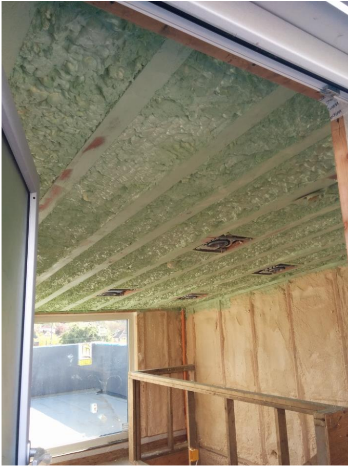
Roof insulation (foam)
