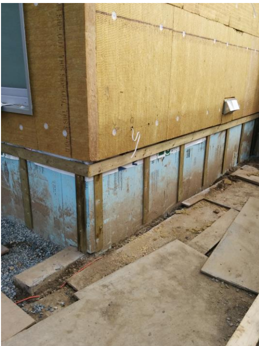
Basement exterior insulation
