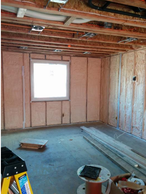
All exterior walls foam and tape
