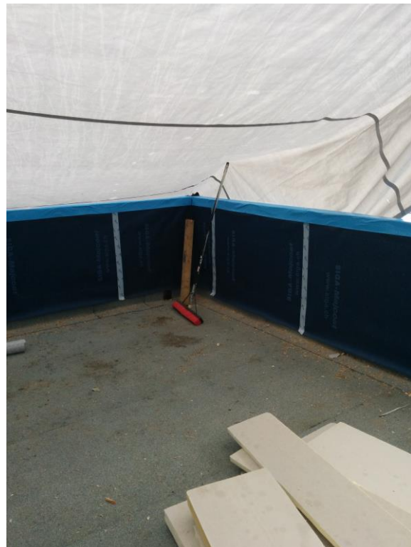
Parapet membrane to roof
