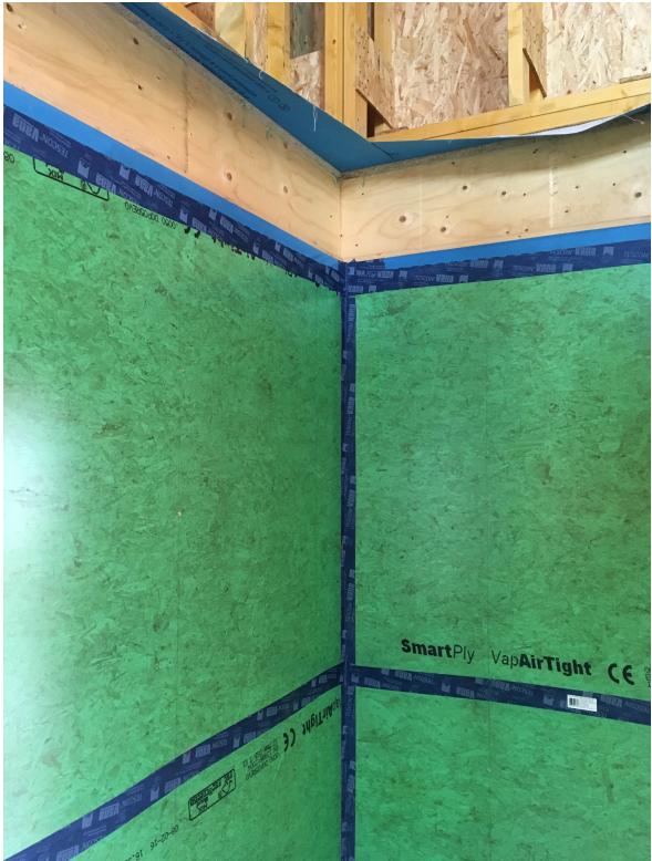
Figure 9, showing taped boards and membrane at floor to floor junction.
