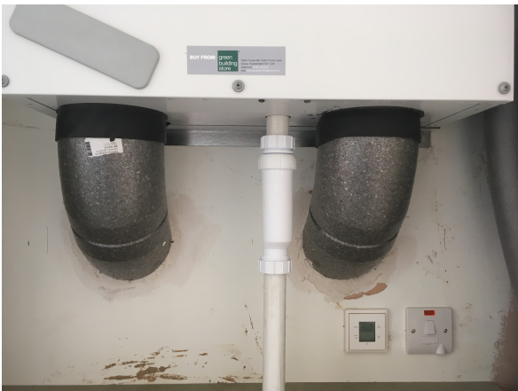
Figure 13, detail of MVHR installation.
