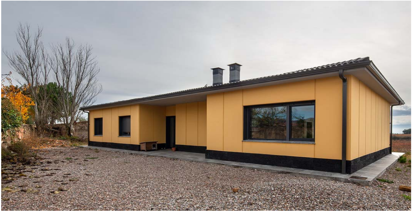
North view, Source: Construcciones Zorzano
