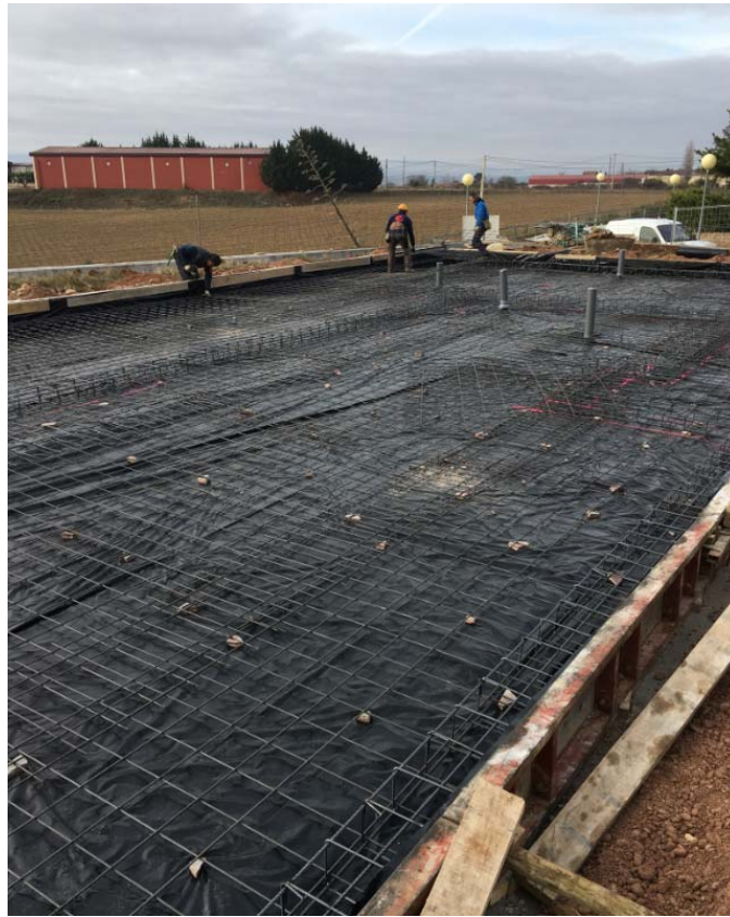
Basement floor (Source: Construcciones Zorzano)
