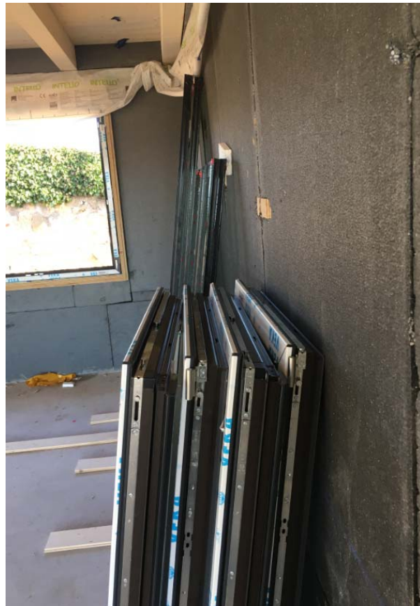
Window installation (Source: Construcciones Zorzano)
