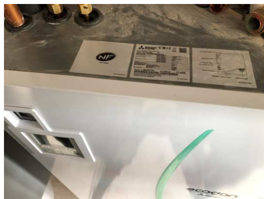
Ecodan Hydrobox (Source: ra[ ]el arquitectura)
