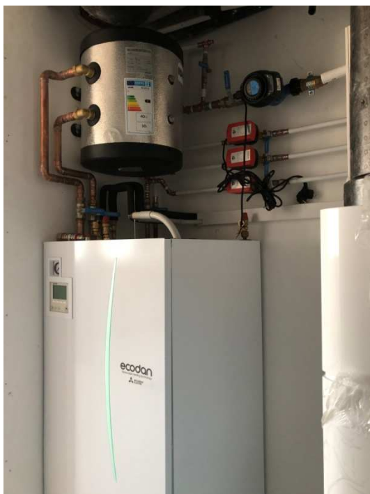
Ecodan Hydrobox (Source: ra[ ]el arquitectura)
