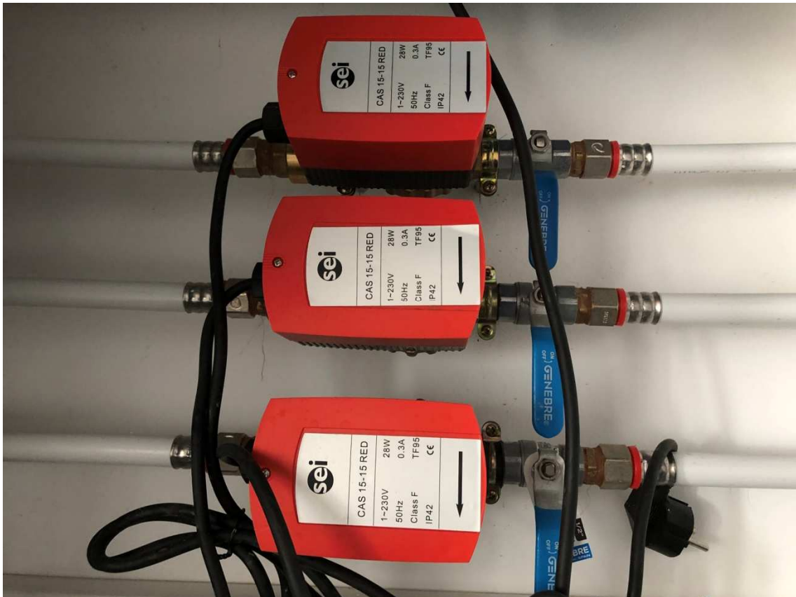
Circulating pump for sanitary hot water (Source: raf jel architectura)
