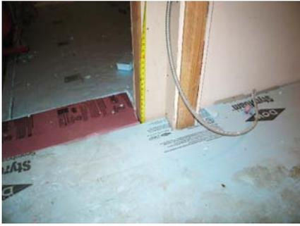
A continuous 3" layer of R5/inch XPS was installed over the new slab throughout the cellar with an additional layer of insulation under the slab where grade beams were not required to reinforce the existing cellar walls. The existing stone walls were air-sealed with Sto Emerald Coat, and taped (with ProClima Vana) to the vapor barrier for continuous air-sealing.
