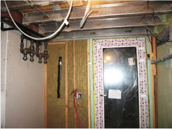
Interior insulation was added to the existing front cellar wall. Insulation was installed continuously and between wood battens which support the finished wall.
