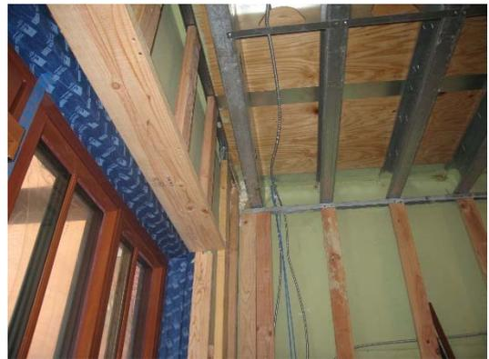
Photo left: step 1 flush air-sealed wall at transition between existing brick and new timber construction. Photo right: step 2 interior (service) cavities upper part of 3rd floor wall- later filled with mineral wool insulation
