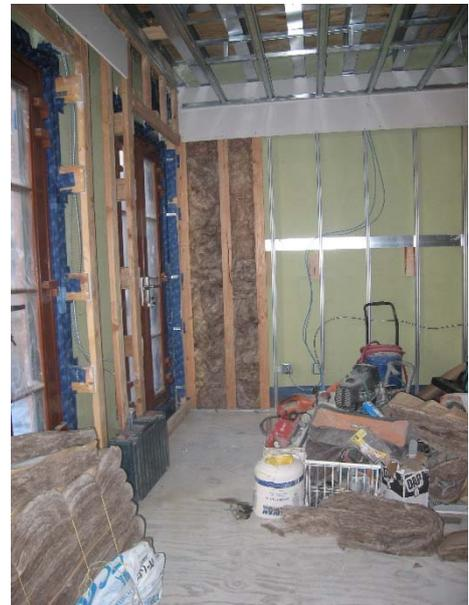
Photo right: 2nd floor party wall insulation and wood battens extend inside 3' min. from exterior exposed front wall. The party wall is adjacent to the neighbor's conditioned space.
