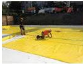
15mil Stego vapor barrier is applied over the entire slab
