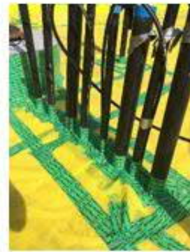
All service penetrations are meticulously taped for state of the art airtightness
