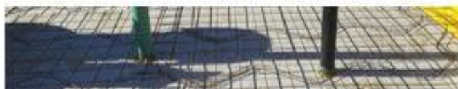
Snake chains and reinforcing steel in place, ready for basement slab concrete pour.
