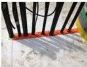
All service penetrations are spray foamed in place
