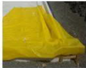
15mil Stego vapor barrier to extend min 12" beyond the edge elements for a future good lap with the foundation wall airtight layer
