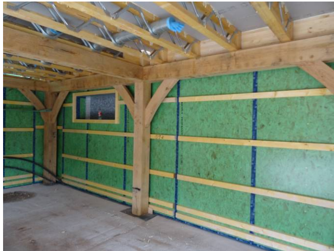
Example of taping of panel joints (void battens left short for ease of taping)
