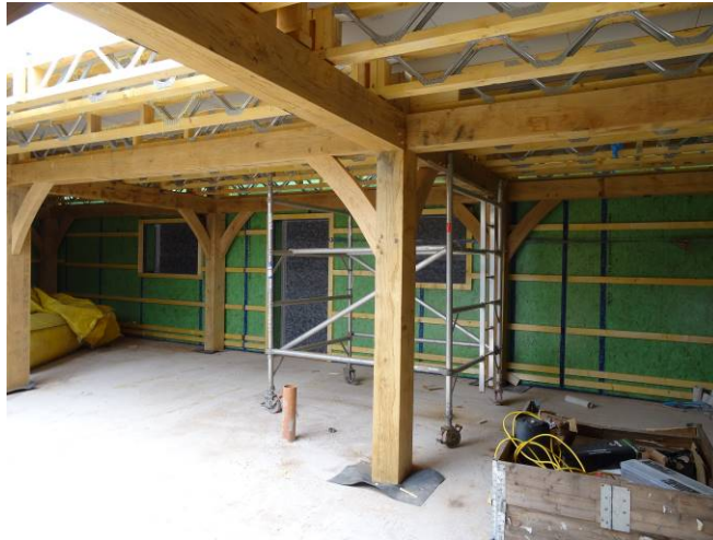
Example showing to green oak frame on RC slab and inboard of airtightness layer
