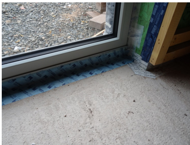
Example of sliding doors sealed to slab prior to pouring of screed
