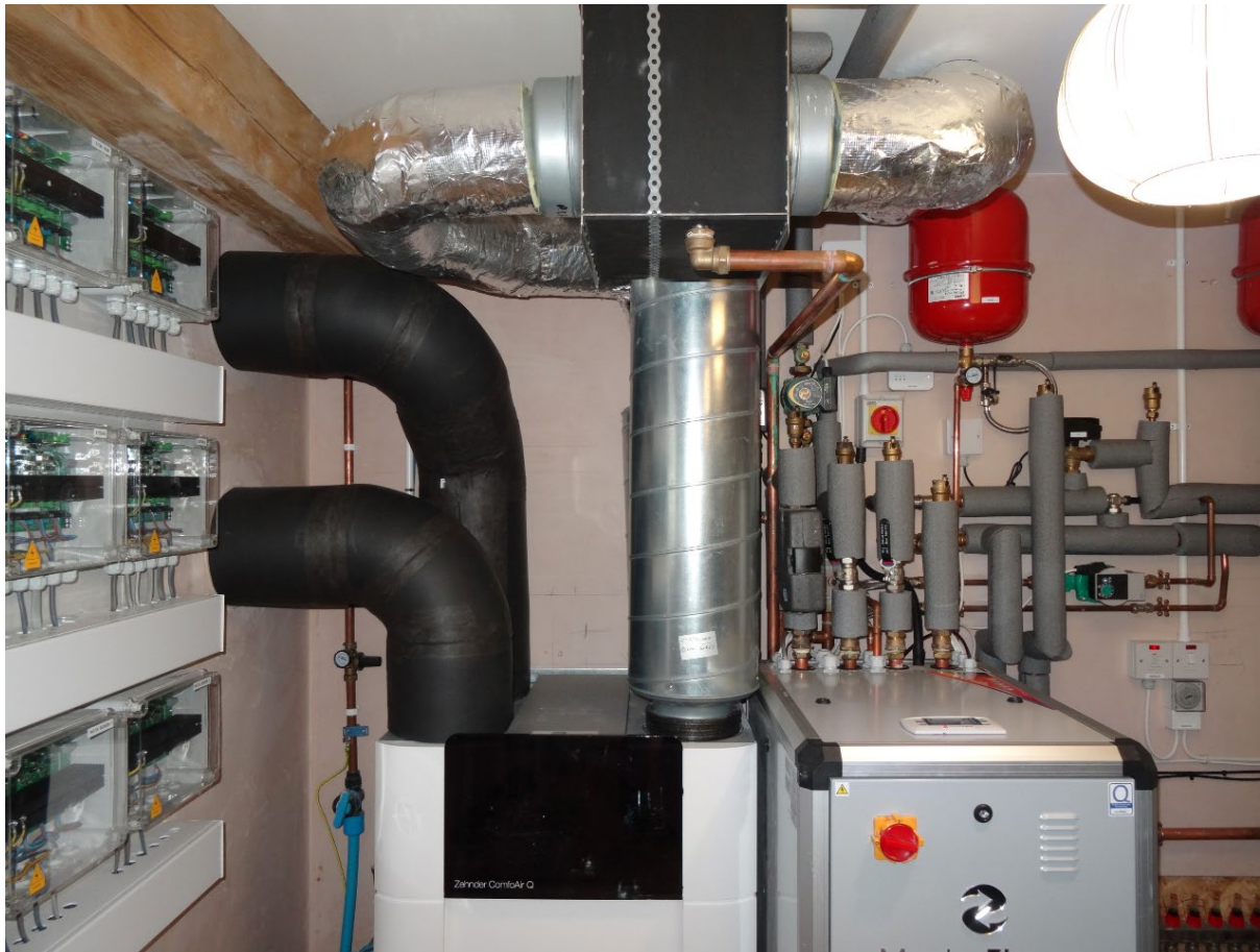
Photo of MVHR installation prior to the cooler battery and feed pipework being insulated
