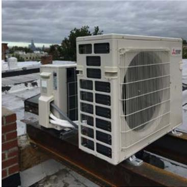
Because of the need for mechanical cooling and dehumidification in summer in New York, ducted heat pumps were selected to supply cooling and dehumidification in summer as well as heating in winter. The ducted indoor units require relatively little space and provide zoned controls for the owners.
