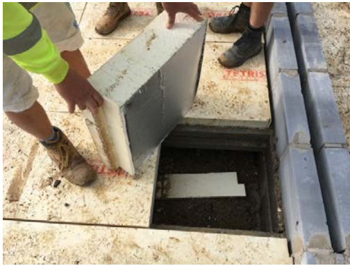
Tetris floor system – photo shows the profile of the insulation block which sits between beams. A second layer of insulation was installed over the top.
