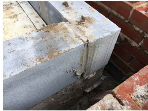
Quinnlite blocks, installed to the perimeter of the floor zone.
