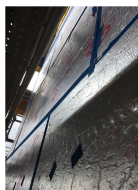
External wall insulation with Weathertightness tape
