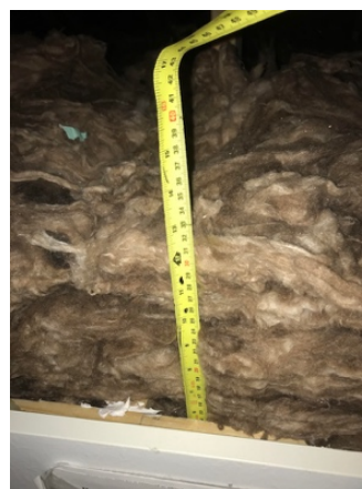
Loft insulation in cold roof space (photo supplied by Drew Smith Ltd)
