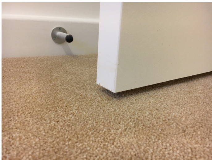
Top left and right: Rigid metal ductwork installed within first floor structural zone. Above left: silencers to the rear of the MVHR unit. Above: Paul unit in cupboard. Door oversized to allow for removal. Left: Undercut to door to allow for air flow. (photo supplied by Drew Smith Ltd)
