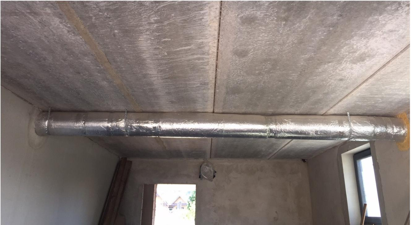
The ventilation duct is designed through the garage space to the outside wall.
