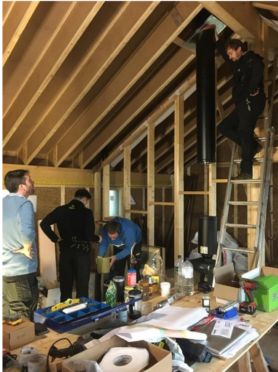
Installation of wood stove and flue
