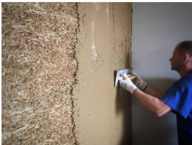
Clay plaster applied to Ecococon straw panels wall
