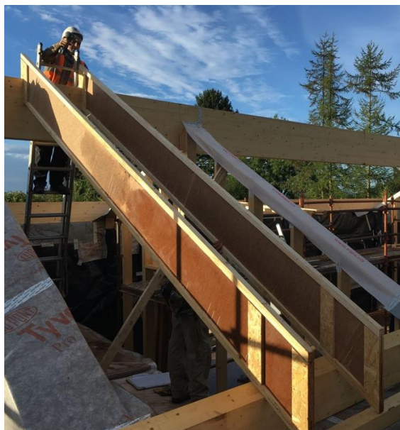
Installation of roof joists
