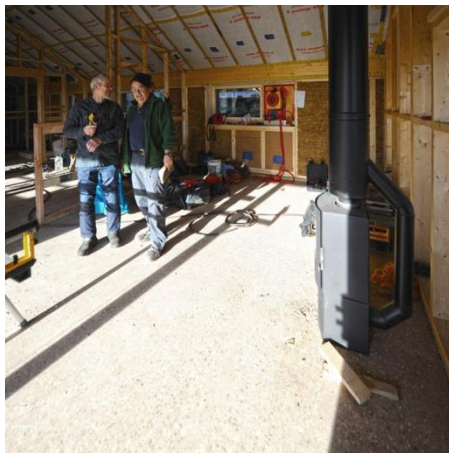
Initial air test with Paul Jennings and Nick Grant. Notice the small fan installed in the window
