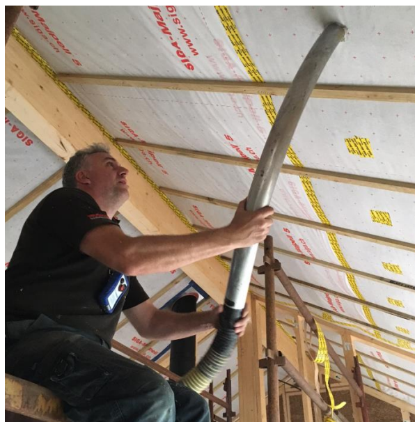
Installation of Warmcel insulation between roof
