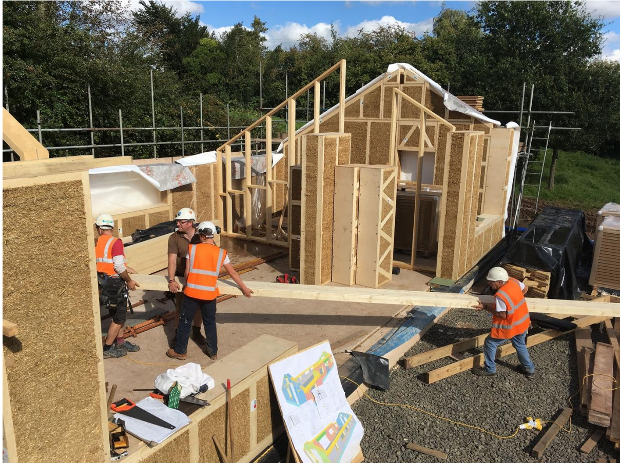
Installation of Ecococon prefabricated timber/ straw wall panels with no heavy machinery needed. All external walls were finished in three days.
