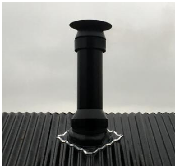
Triple wall flue roof terminal with integral air intake and exhaust
