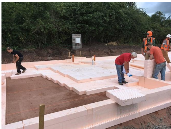
Installation of Isoquick EPS foundation insulation
