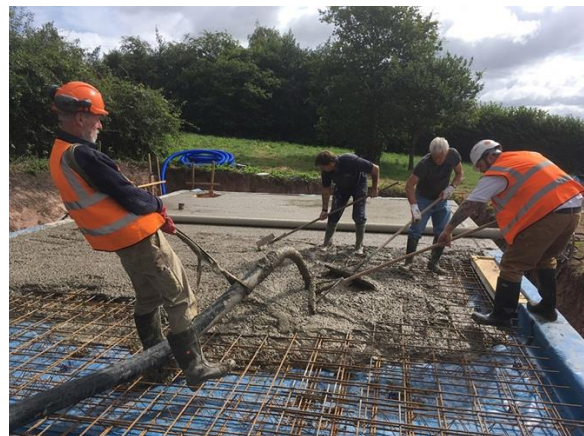
Pouring of concrete slab
