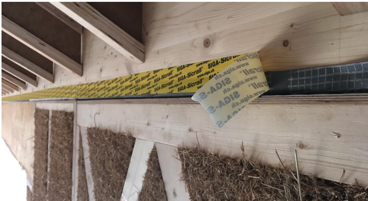
Airtightness membrane sealed to glulam wall plate, before airtightness membrane was installed under roof timber I-beams
