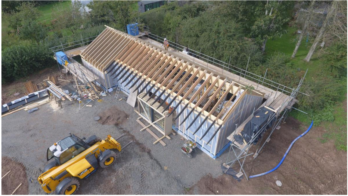
Aerial view of the construction site showing the walls (before woodfibre installation) and roof elements
