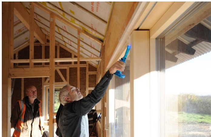
Nick Grant checking for air leaks using smoke gun
