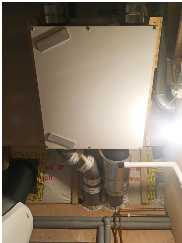
Ceiling mounted MVHR unit
