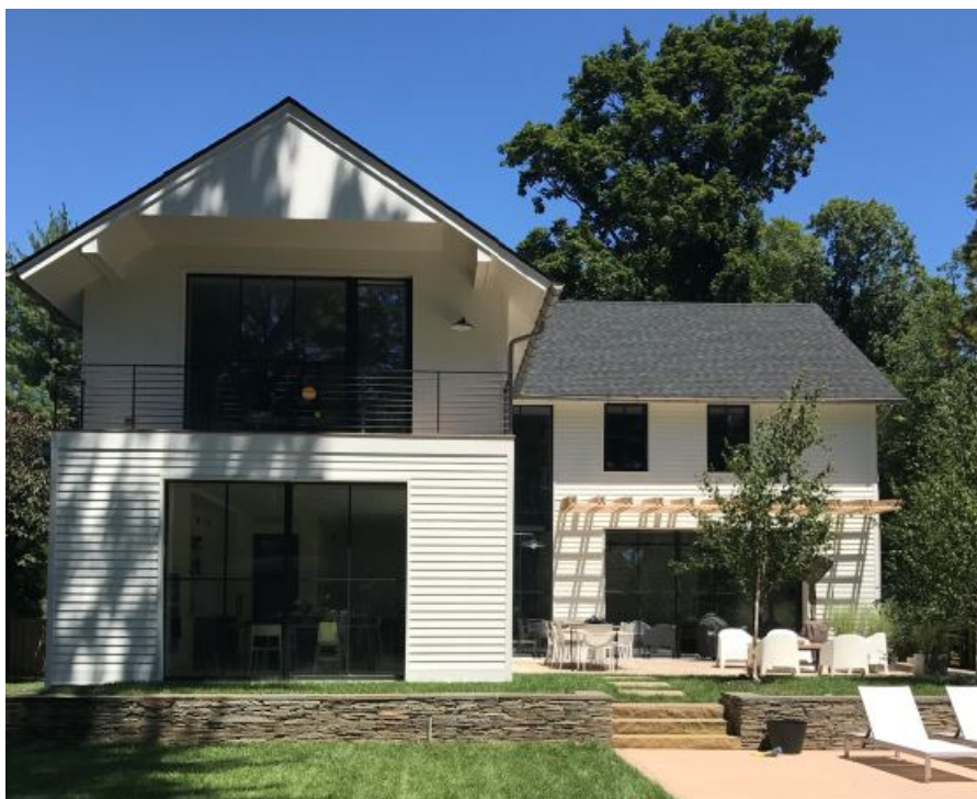
Single family home with two floors and full basement in Madison, New Jersey
