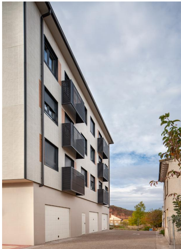
North view Source: Construcciones Zorzano
