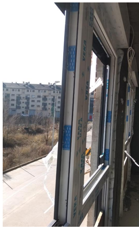
Window installation (Source: Construcciones Zorzano)
