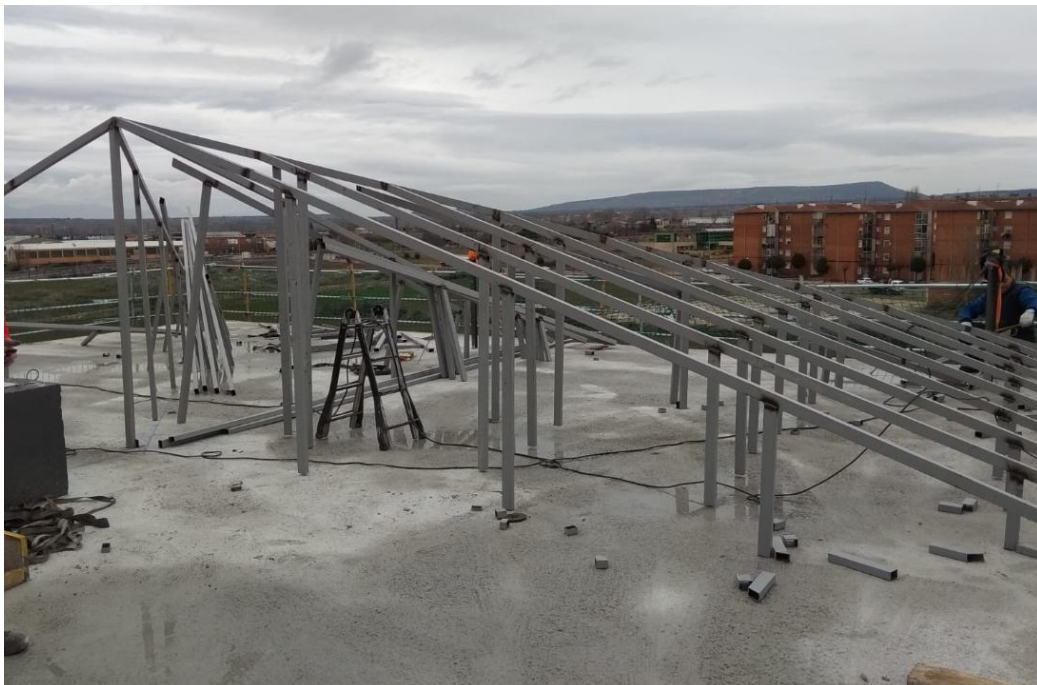
Structure cover building (Source: Construcciones Zorzano)
