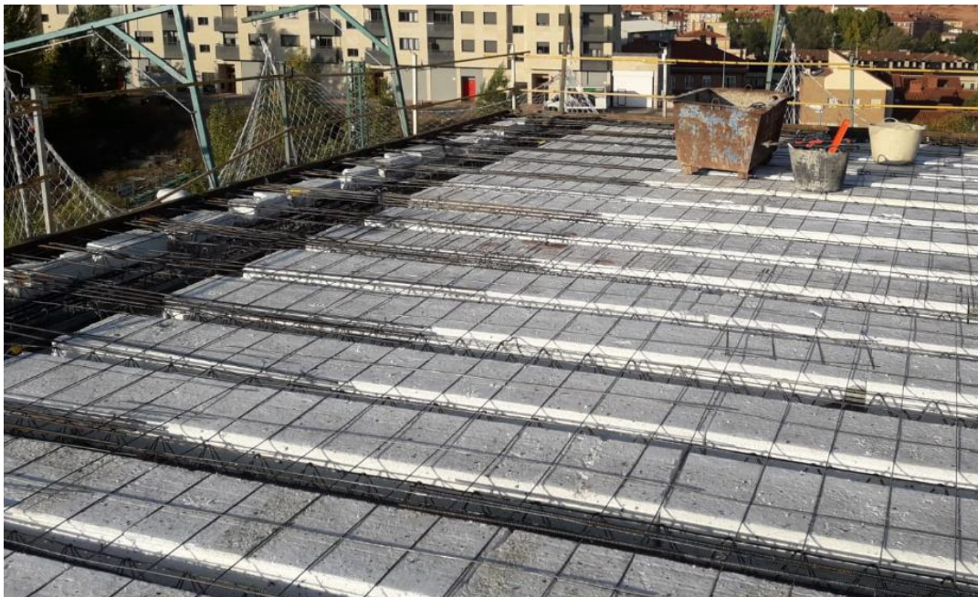
Basement floor (Source: Construcciones Zorzano)
