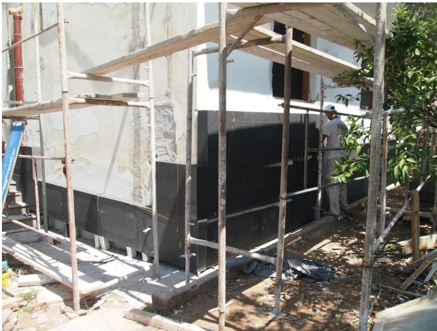
Picture 8. Placement of the exterior insulation of the thermal envelope
