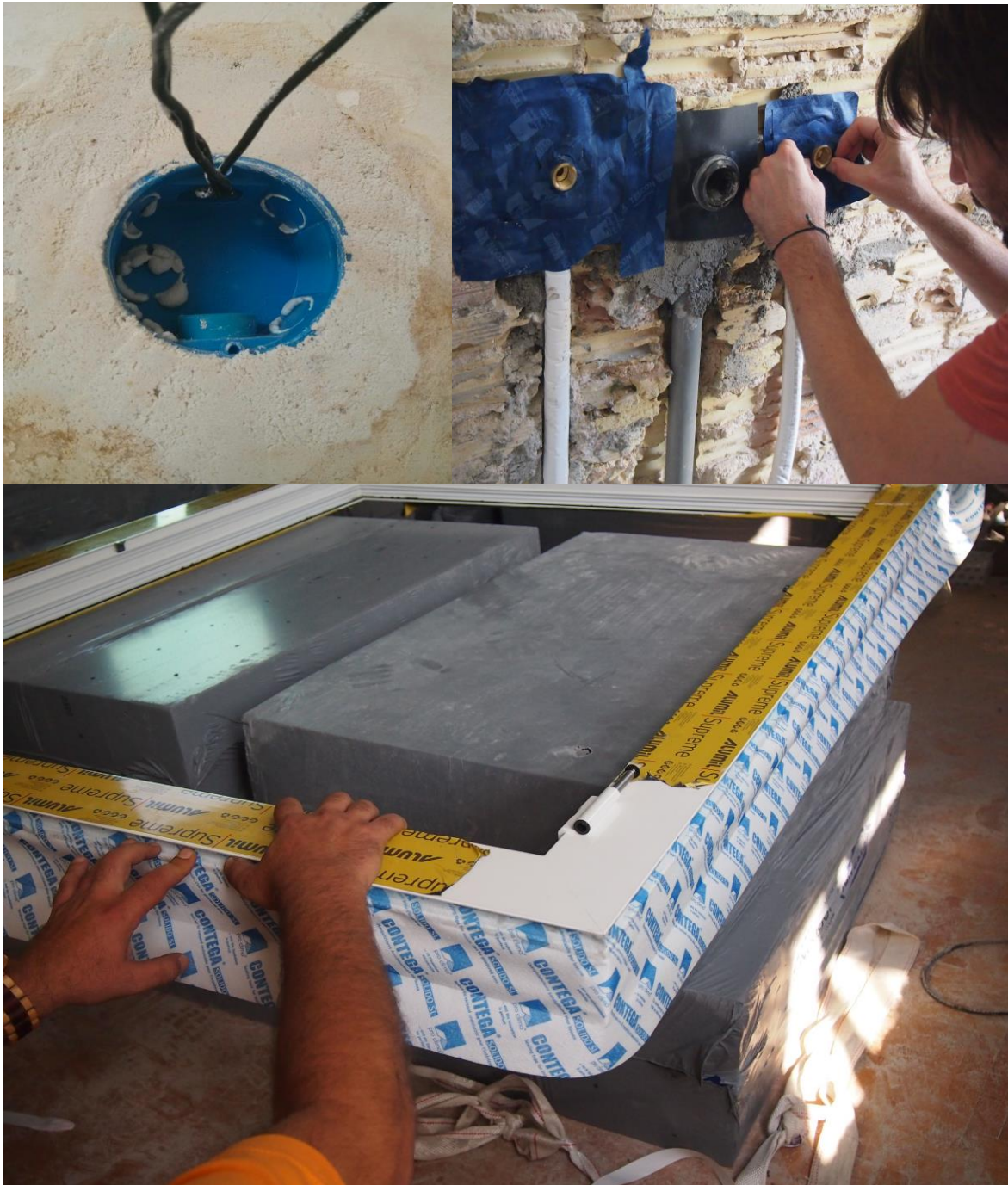
Picture 14. Airtightness measures in window installation
